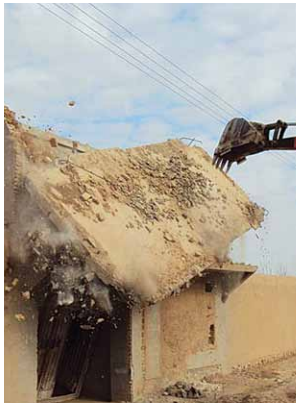
Homes being destroyed to widen road, Khulm
