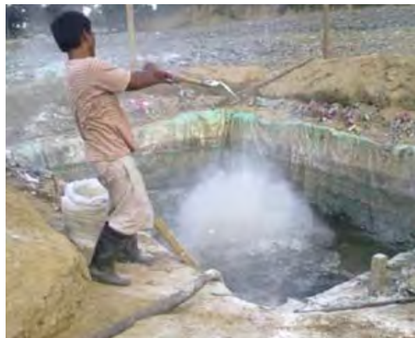
Figure 25 Spraying of hydrated lime on sludge/Photo courtesy of HRC
