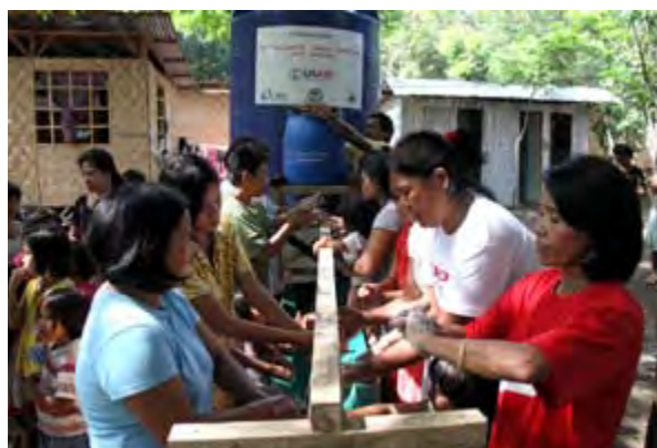
Figure 20 Group handwashing stations made out of GI sheets and coco lumber in TS/Photo by Jen Hardy for CRS
