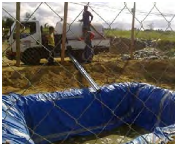
Figure 25 Spraying of hydrated lime on sludge/Photo courtesy of HRC
