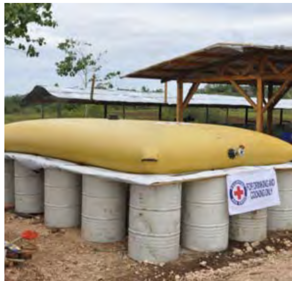
Figure 6 PRC Bladder with Oil Drum and Plywood Bladder Stand/Photo by Kate Davis
