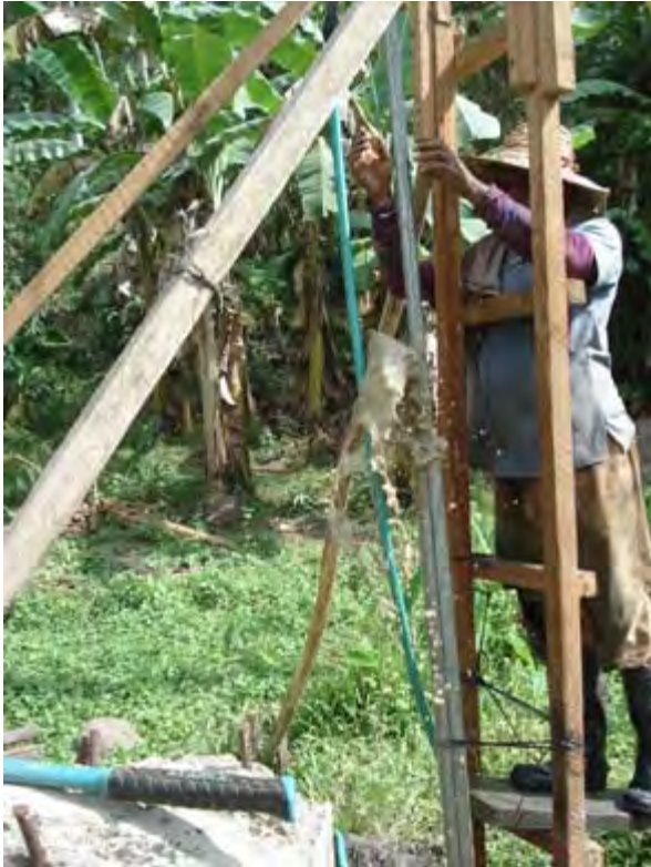
Figure 11 Sludger drilling/Photo by Nyunt Lwin
