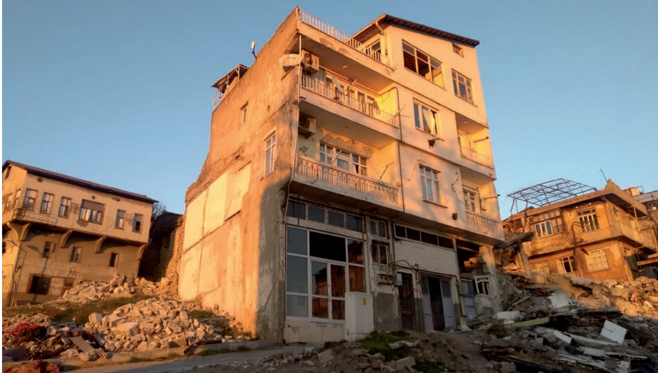
A building standing in the middle of rubble, in Kahramanmaraş, one of the areas where networks were impacted the most. ©Photo: Télécoms Sans Frontières
