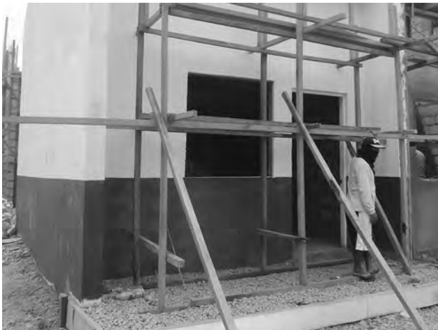
Figure 9. Permanent row house with walking loft designed by NHA and built by GK in Tanauan, Leyte. Photo: by the author, March 11, 2014
