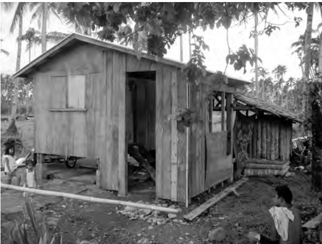
Figure 5. Temporary coco lumber and wood shelter, elevated 0.90m above the plot; a self-built extension at the back of the house is used as a covered kitchen. Javier, Leyte. Photo: by the author, March 10, 2014.
