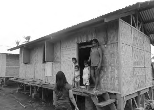
Figure 6. Temporary shelter made with amakan, traditional woven bamboo wall, elevated 0.80m above the plot, provided by CRS in Caparas an Guti, Palo, Leyte. Photo: by the author, March 13, 2014.
