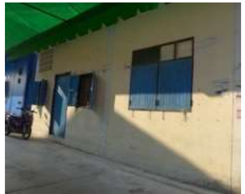
Single storey cement homes
