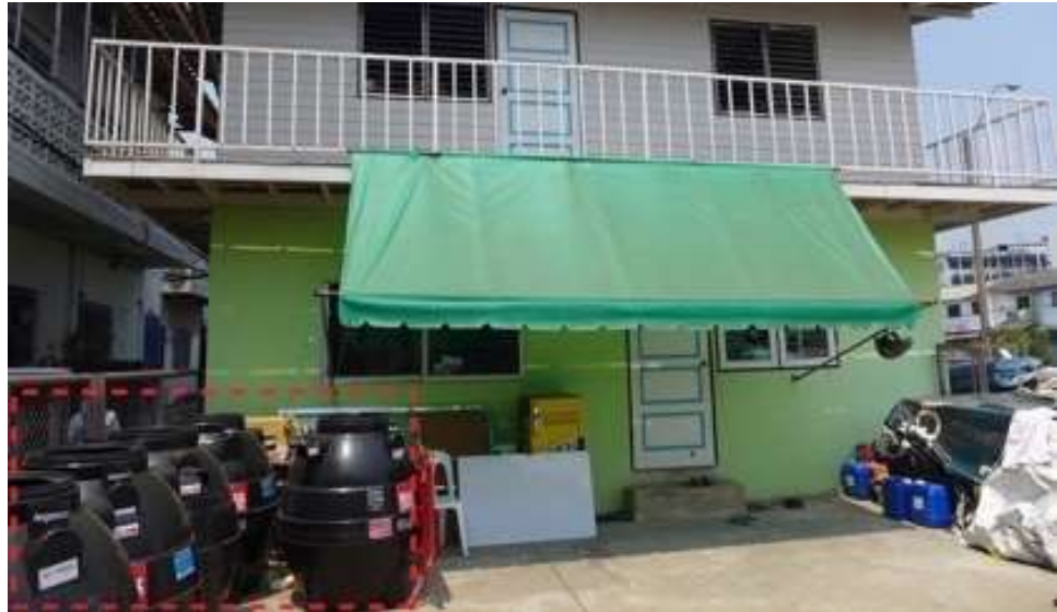
Figure 8.5.2a: Sewerage tanks pictured in front of the community building are fitted into the newly reconstructed homes. Source: the author
