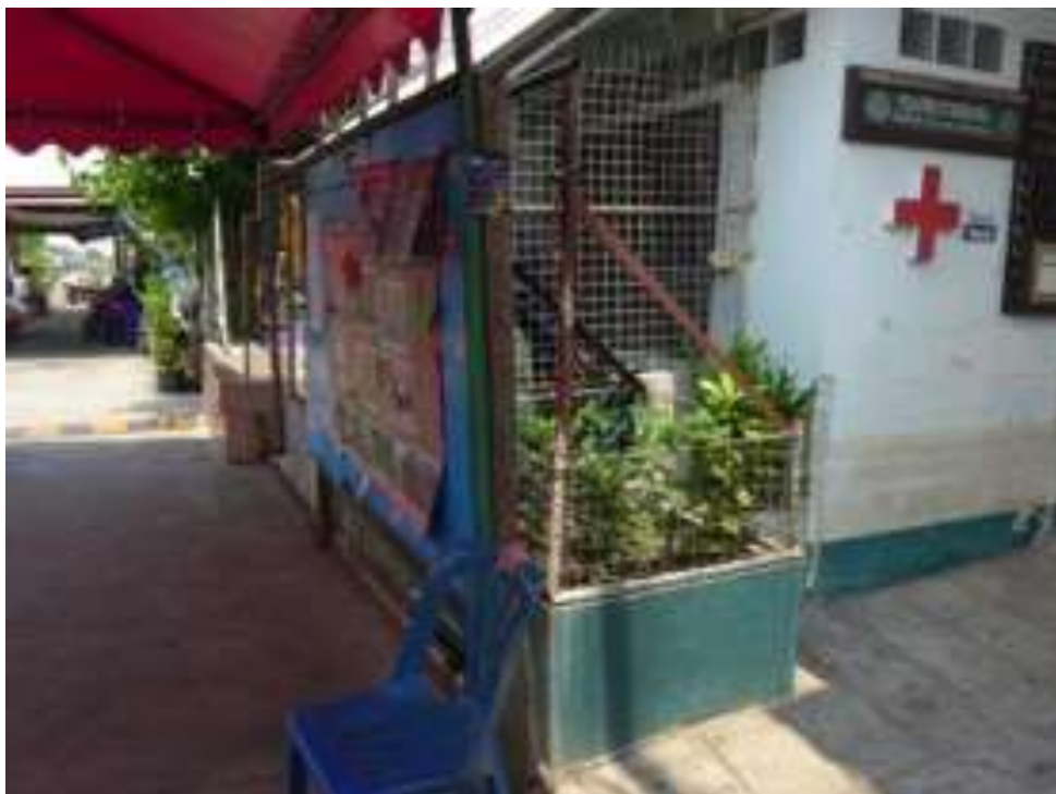
Figure 5.4.1c: A health centre a few hundred metres from Bang Bua Neighbourhood. The clinic is a single storey building made of cement. Source: the author
