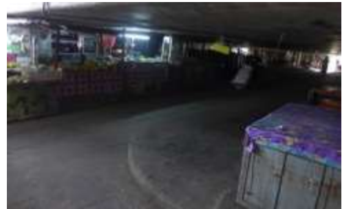
Pedestrian lane under Phaholyothin Rd. bridge (case 3)
