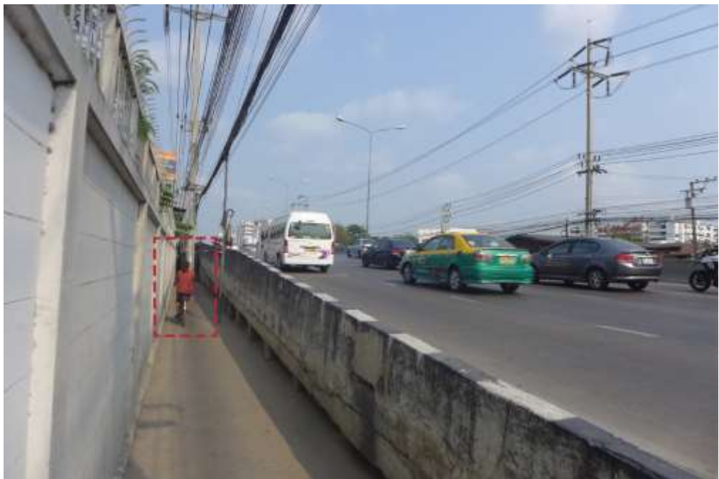
Figure 9.3.1d: Access to Roi Krong is gained through a narrow lane that runs parallel to the bridge incline. Source: the author
