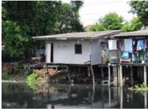
Single storey wooden stilt homes
