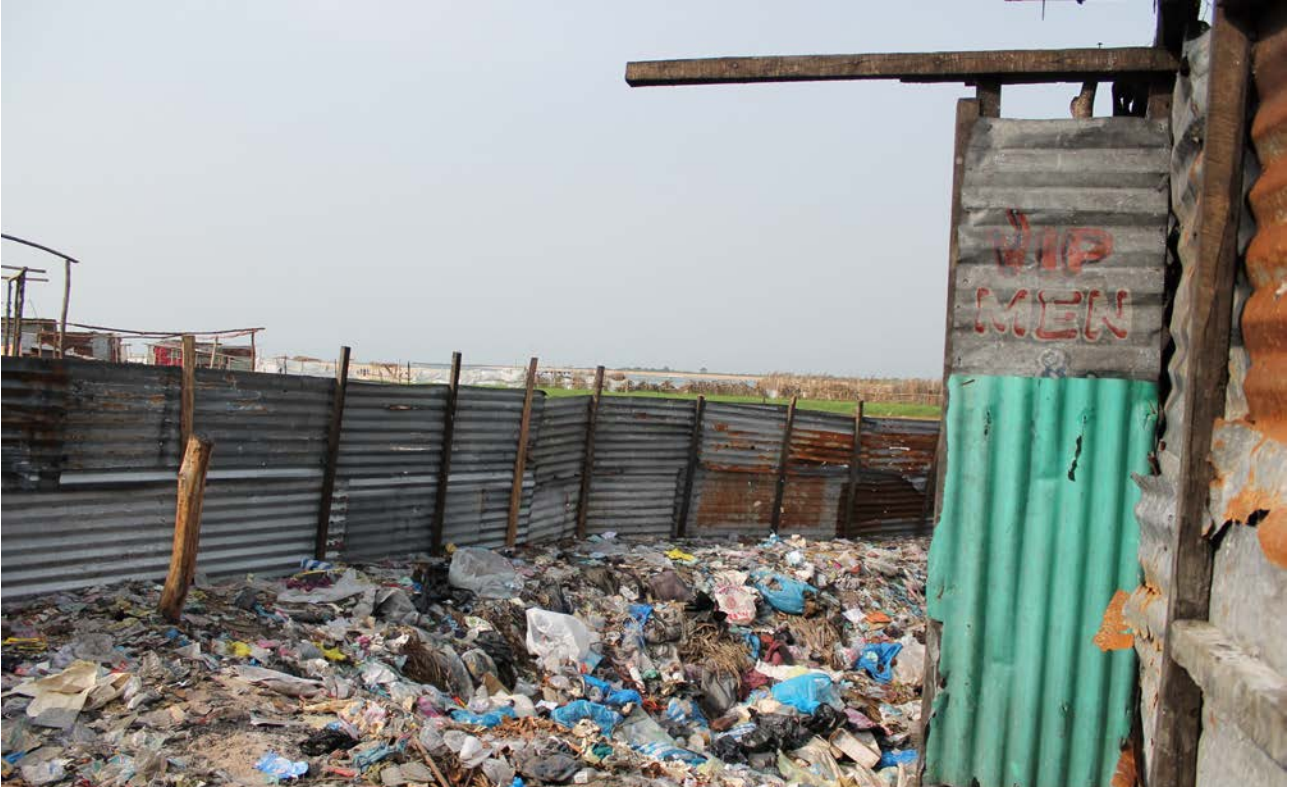
A makeshift and poorly constructed latrine built in West Point
