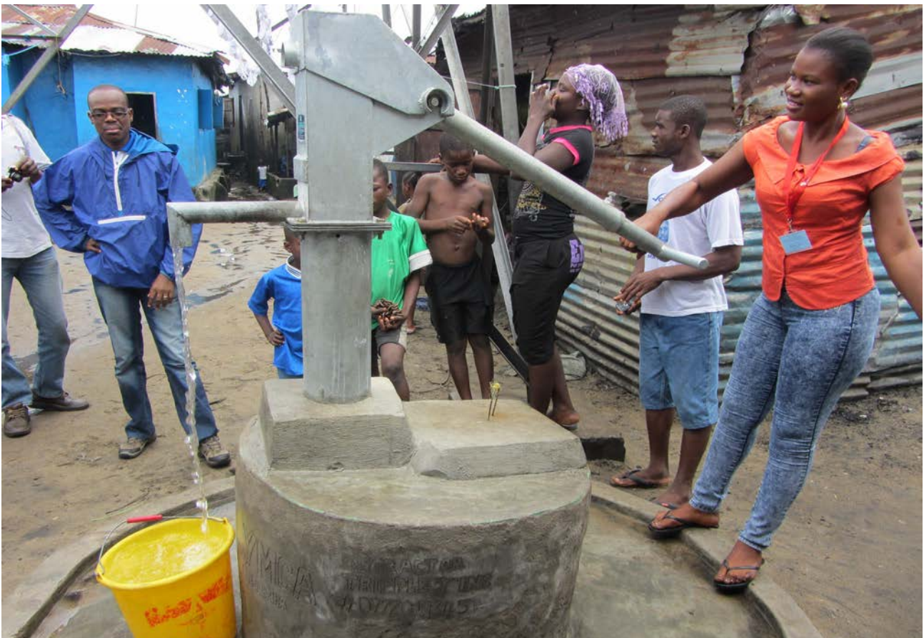
A water point constructed by the YMCA in West Point
