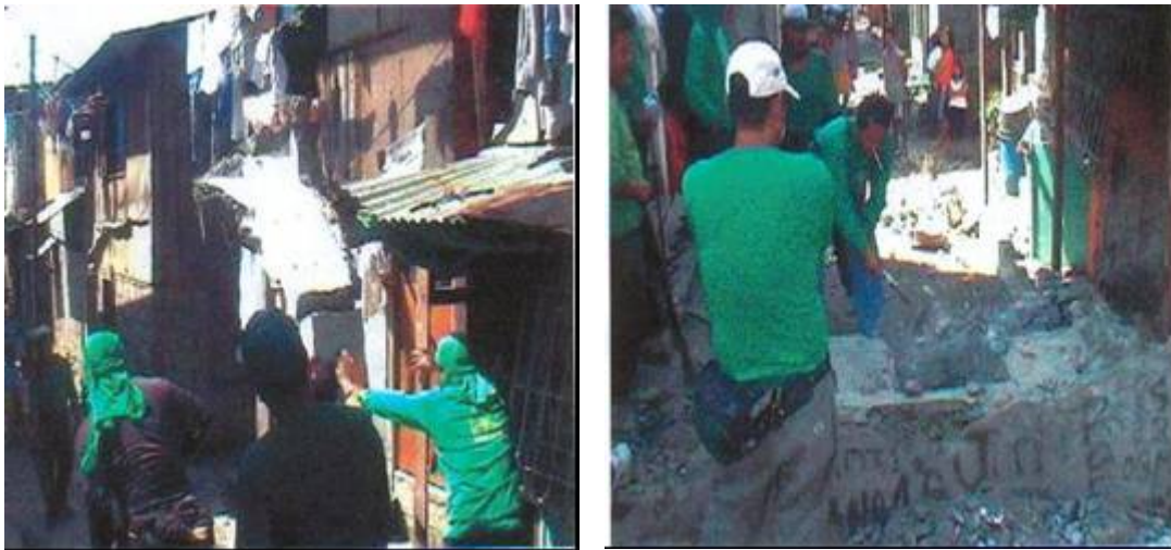
Marikina's demolition team in action
