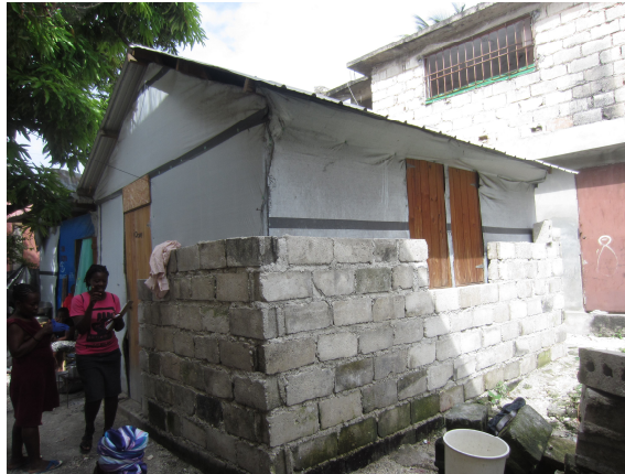
Figure 5 Incremental development to a humanitarian T-shelter.
