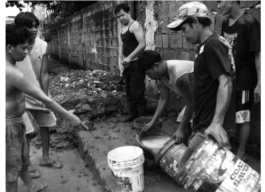
Community members widen the exit route by the riprap.
