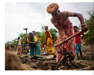
During the two dry seasons (from January to June), protective and productive infrastructure is rehabilitated under the technical guidance of LGED, using unskilled labour of the ultra-poor, largely women. The embankments, road cum embankments and canal infrastructures are intended to reduce the negative impacts of climate change effects and prevent flooding and tidal surges; and to facilitate drainage during the monsoon and irrigation water during the dry season.
