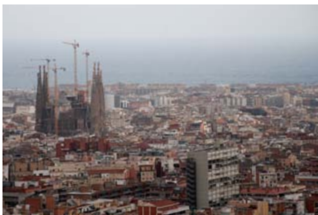
The city of Barcelona is working on resilient infrastructure through its Infrastructure Urban Resilience Board (TISU)
