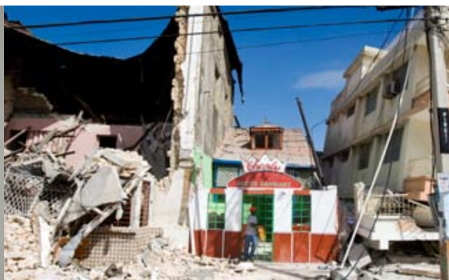
Destruction in Port-au-Prince, Haiti, after the magnitude 7.0 earthquake in January 2010.
