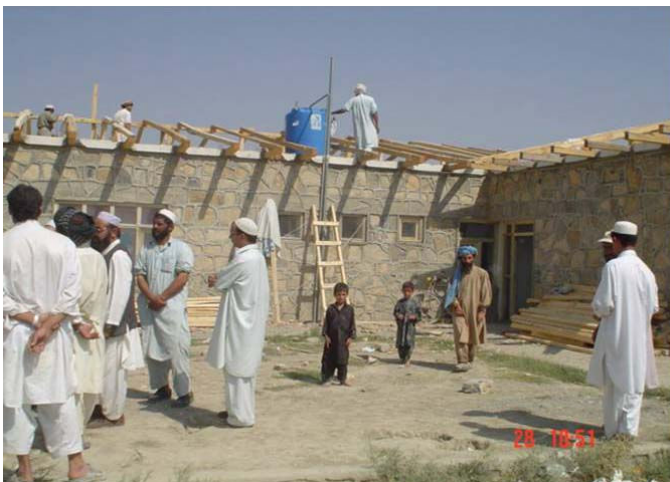
Construction of a clinic in Khost Province
