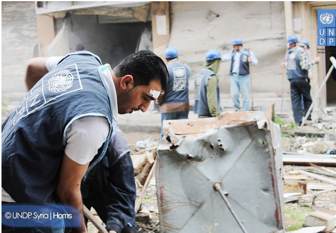
UNDP workers clear rubble from depopulated Old City neighborhoods in Homs
