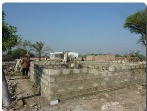
Illustration 5: Construction work at TMK site
