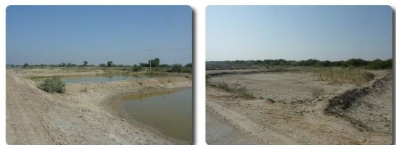
Illustration 8: Damaged and destroyed fish-farm ponds, lower Sindh
