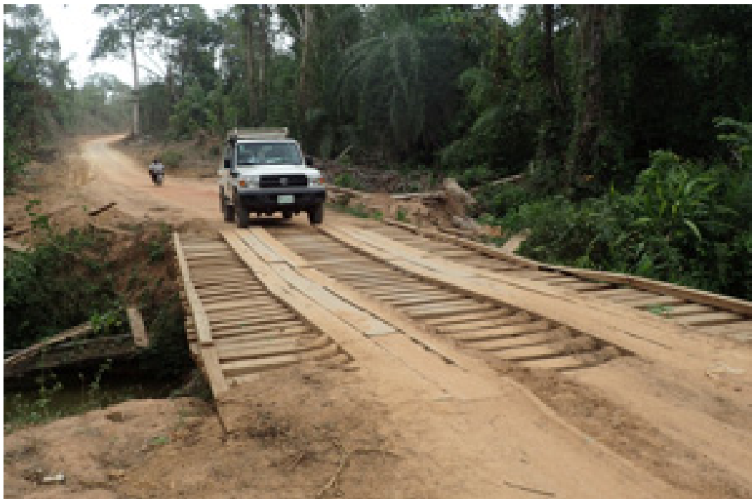
Nimba County, 20 March 2014. Bridge built by Oxfam. Photo: A. Lloyd,/Oxfam
