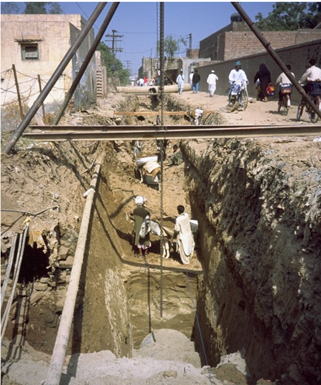
A community sewerage project in Pakistan.
