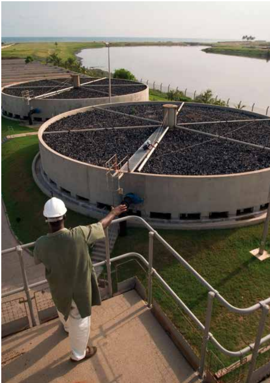
Well-functioning water operators are essential for the delivery of services like this sewage treatment works.
