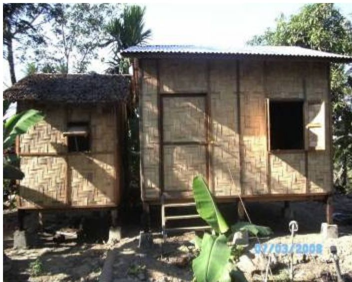
A house and side kitchen built
