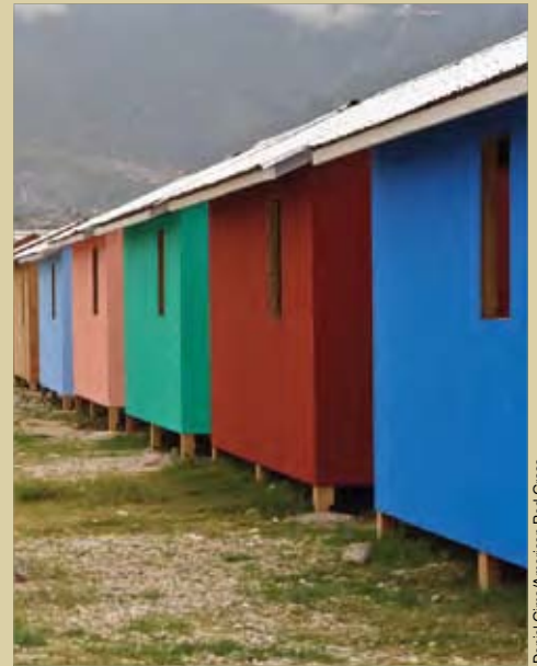
Completed Red Cross transitional homes in La Piste, Port-au-Prince.
