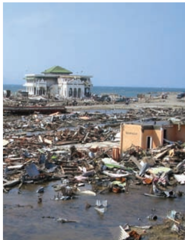
DAMAGE IN BANDA ACEH
