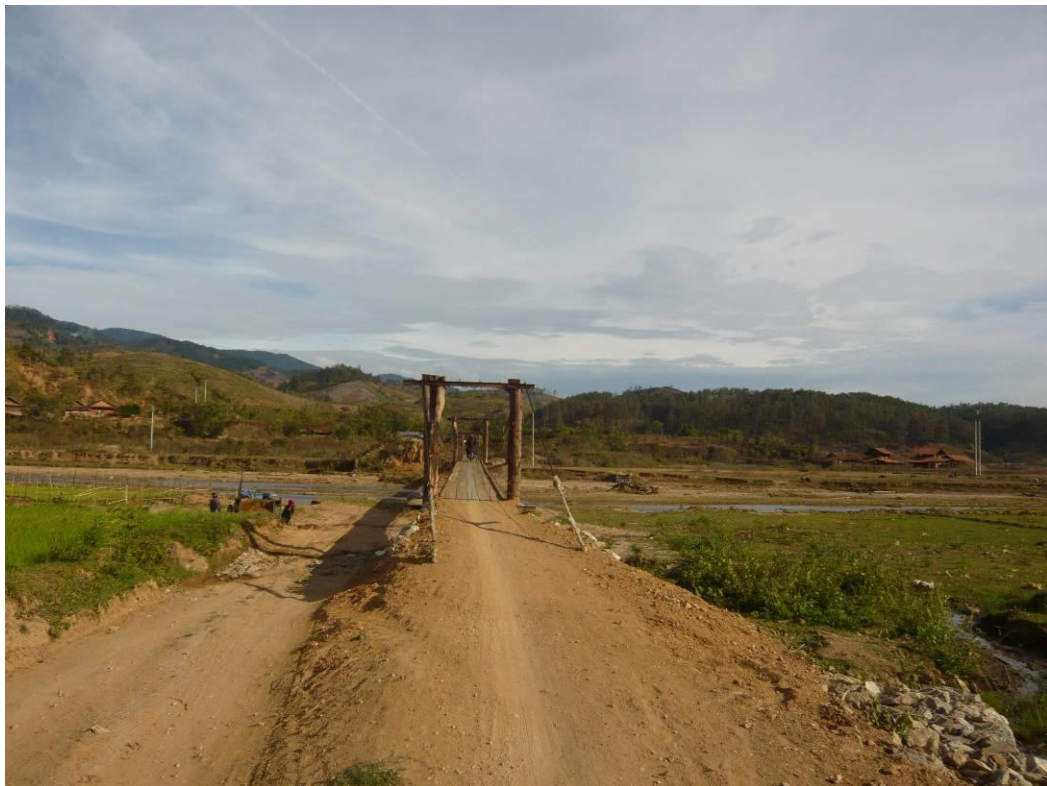
The bridge in Dak Ven, Dak Pet commune – C4W support output
