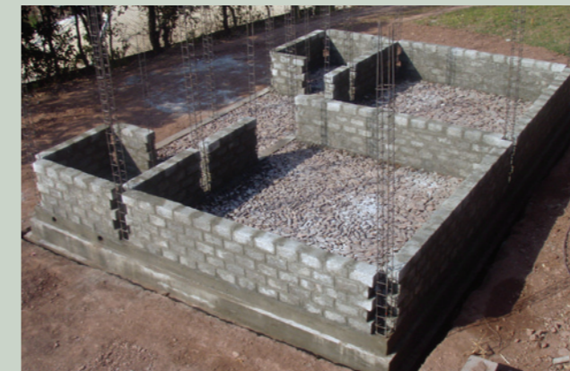
Confined masonry block construction, demonstration house
