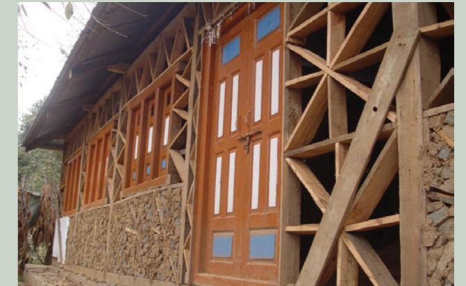
Masonry infilled timber frame, local techniques regenerated
