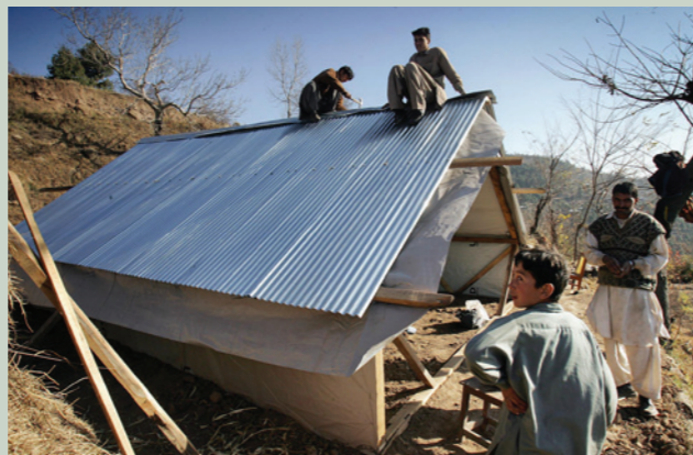
Constructing demonstration shelter, 2005.
