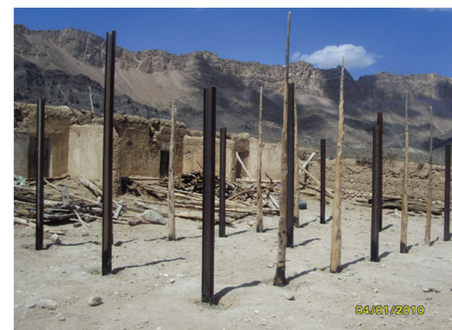
2010, New construction with steel girders to reinforce walls
