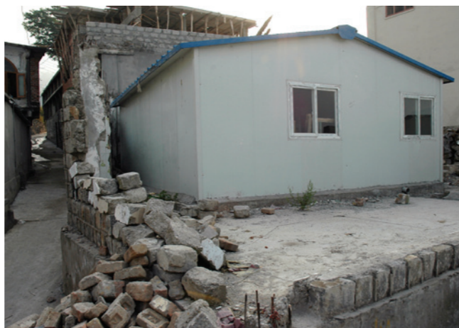
Prefabricated shelter on the site of a 3 storey house, 2008
