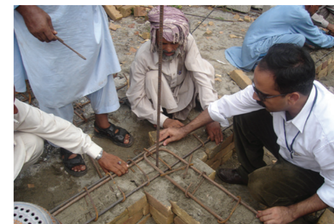
Ahsan explaining reinforcement details with masons
