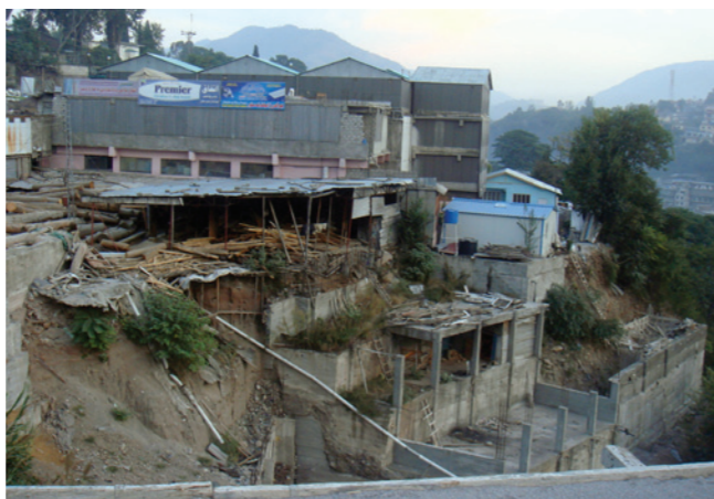
Uncontrolled development in Muzaffarabad, urbanization on marginal land, poor construction quality, increasing risk.
