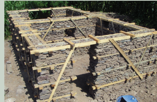
Timber reinforced masonry construction
