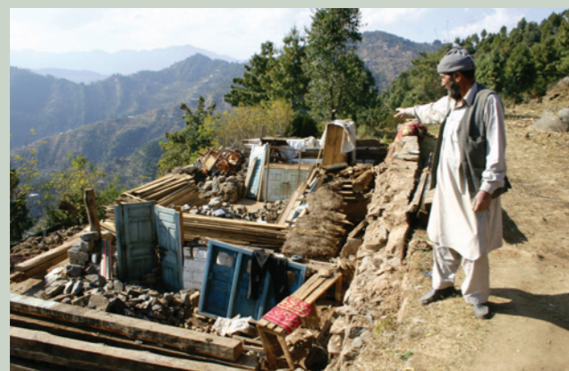
Narrow terraces, many houses include retaining walls.
