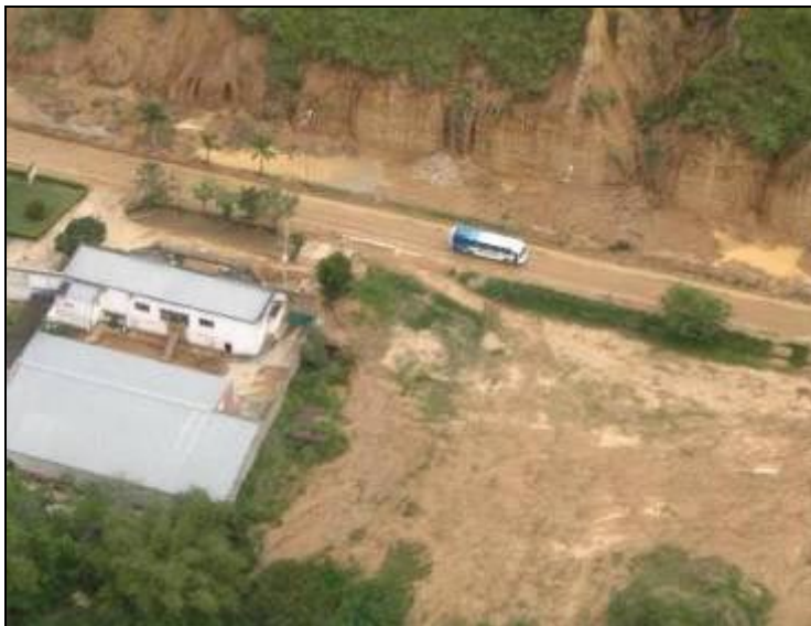
Figure 14. Debris flow in Bucaramanga (Castro 2005).
