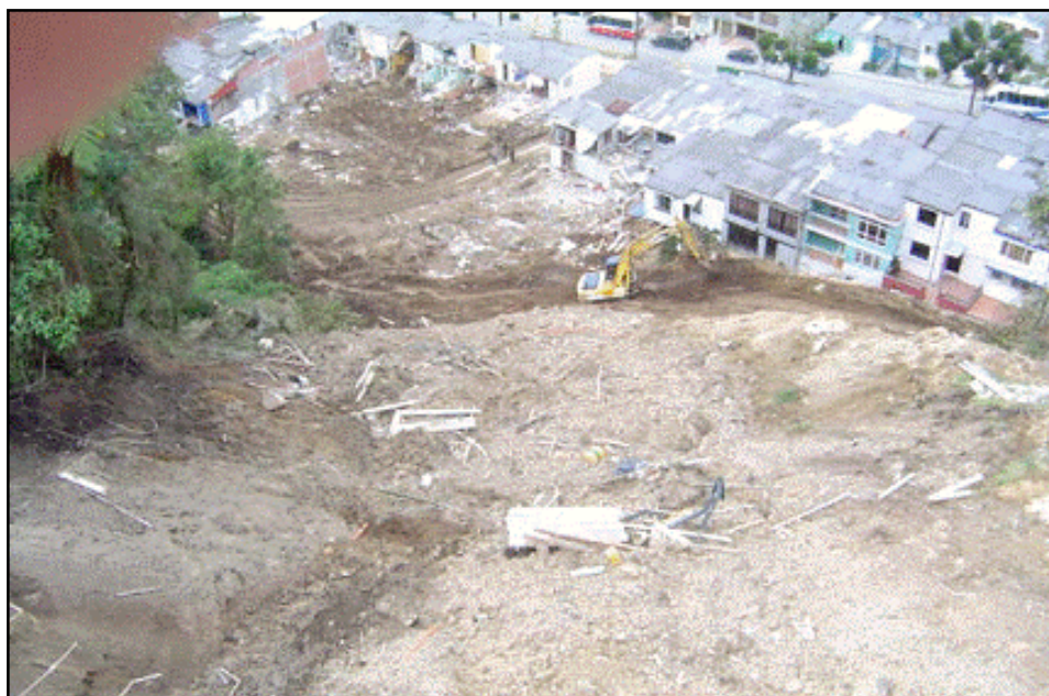
Figure 8. La Sultana (Manizales) landslide looking down slope (Photograph: R. Mendez)
