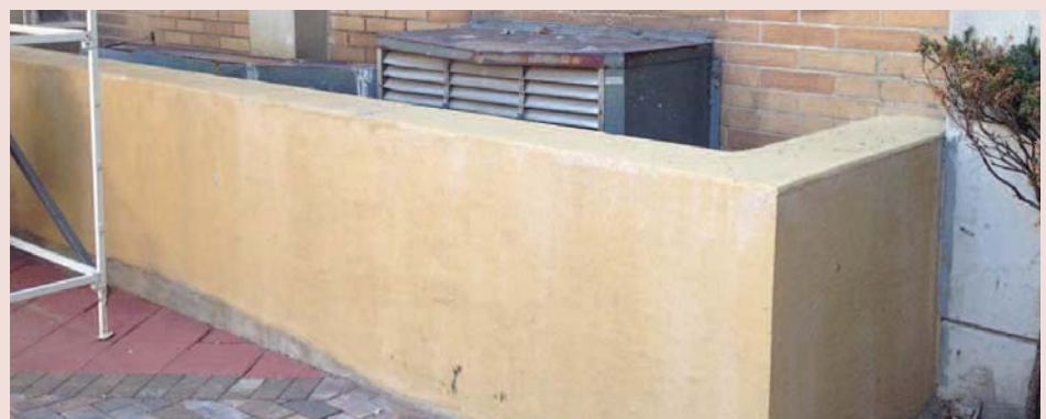
At Shore View Nursing Home in Brighton Beach, a cement wall protects vents for boilers and chillers from over 5 feet of storm surge.
