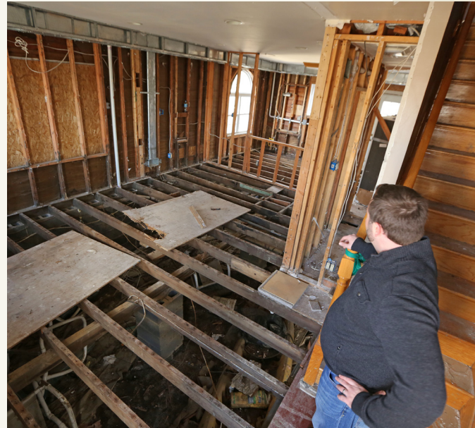
A home in Old Bridge Township, New Jersey, is stripped to the framing for cleanup and repairs. © Frank Conlon/Star-Ledger/Corbis
