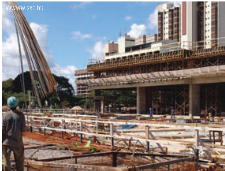
Urban construction site
