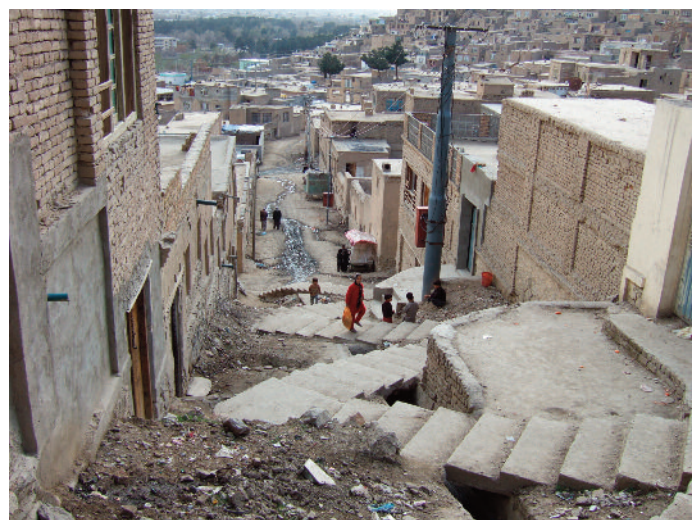
Kabul: construction of an access stairway in the informal zone
