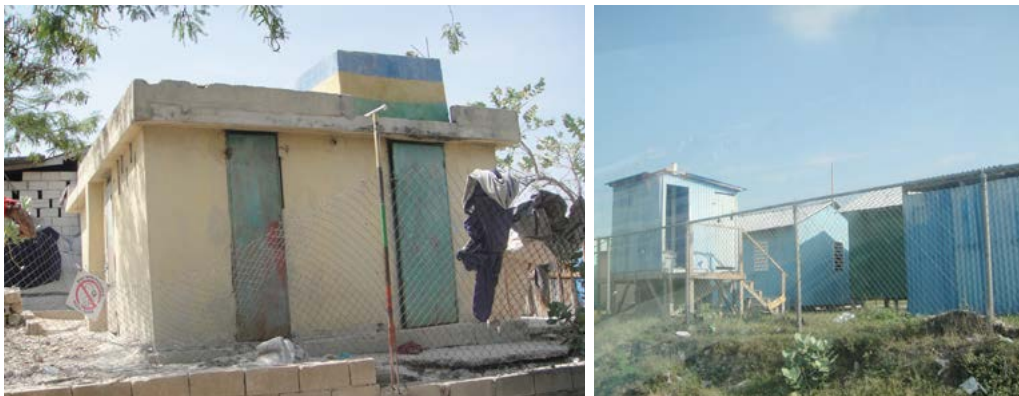
Figure 30. Examples of sewage systems in Haiti camps
