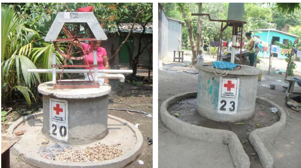
Figure 21. Water wells construction and rehabilitation in El Salvador TD12-E
