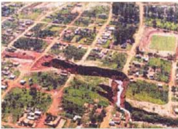
Figure 3.6. Erosion of unprotected urban area (Campana, 2004)
