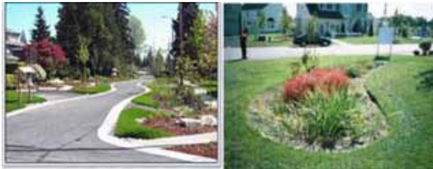
Figure 3.24. The photo (left) shows a street without a kerb allowing part of the runoff to infiltrate into the grass alongside. The photo (right) depicts an infiltration area in a flower bed.
