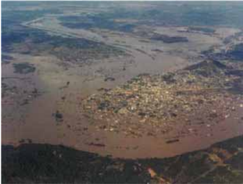
Figure 6.3. União da Vitória and Porto União during the 1983 flood
