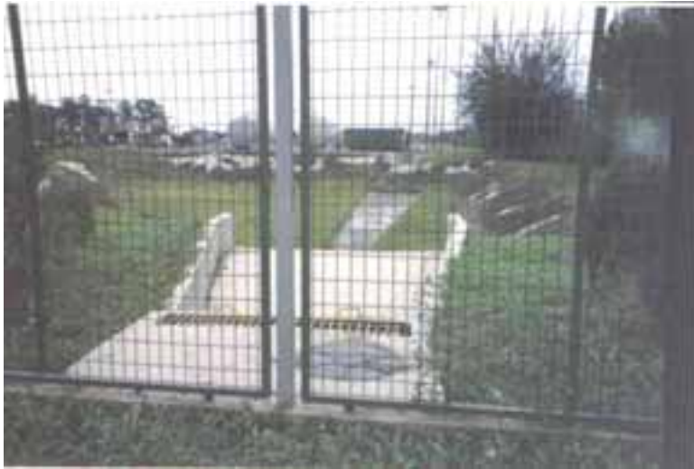
Figure 6.22. Detention basin built for a private project. Córdoba, Argentina (Source: Toya et al. , 2003).
