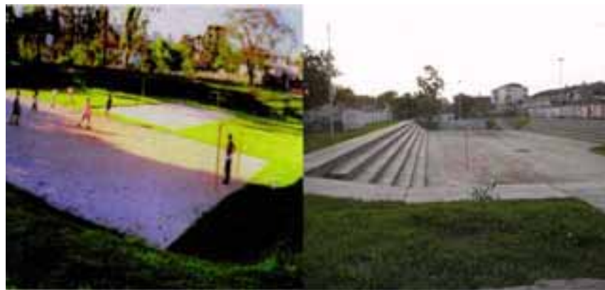
Figure 3.35. Detention basins used as sports fields in Curitiba (left) and Porto Alegre (right)
