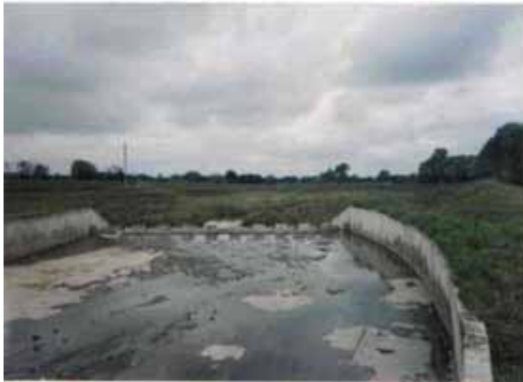
Figure 6.24. Large detention basin built by the public sector.
