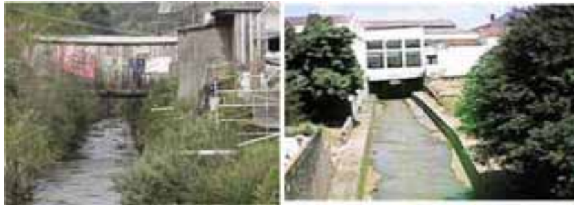
Figure 3.10. Building in drainage channels (Caxias do Sul, Brazil)
