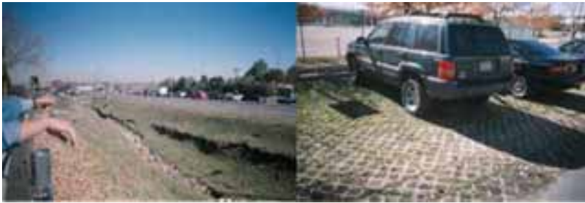
Figure 3.23. The photos show (left) an example of infiltration trenches and (right) pervious paving with perforated blocks for car parking
