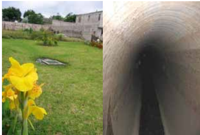
a. View of one of the access chambers to the regulator.
