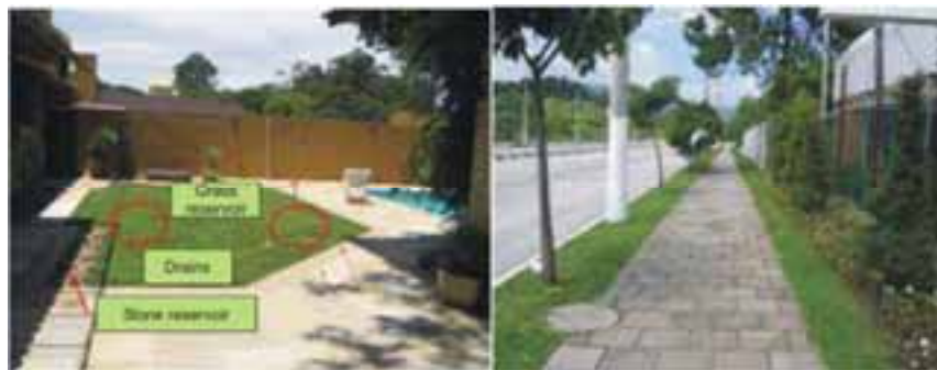
Figure 3.22. Use of systems for retaining water from impervious areas (a) the left-hand photo shows drainage from paved areas onto grass and from roofs into gravel reservoirs; (b) paths with grass alongside to increase infiltration.
