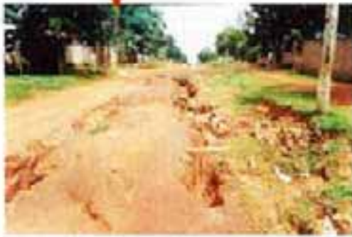
Figure 3.5. Erosion of unprotected urban area (Campana, 2004)
