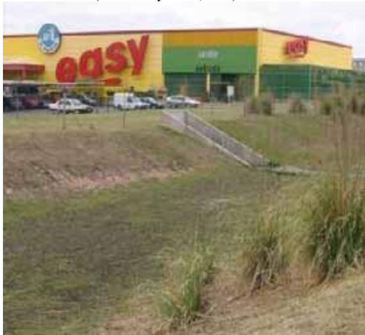
Figure 6.23. Detention basin built for a private commercial project. Córdoba, Argentina (Source: Toya et al. , 2003).
