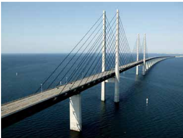
Öresund Bridge, which links Denmark and Sweden and serves as the main entry route for refugees into Sweden.
