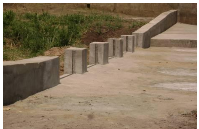
Figure 1 : Kwisa weir before and after rehabilitation
