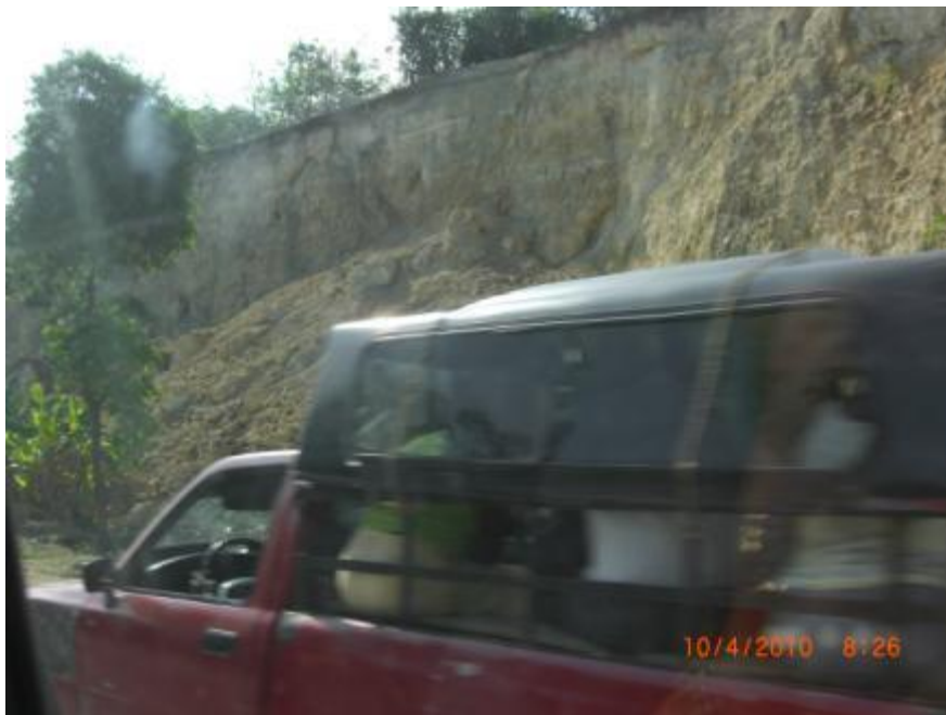
Figure 5.3: A substantial landslide next to the highway
