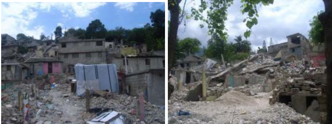
Figure 6.19: Heavily damaged buildings in the area immediately to the south of location 17.
