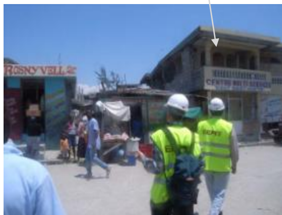
Figure 6.12: Ground view of building (b)
