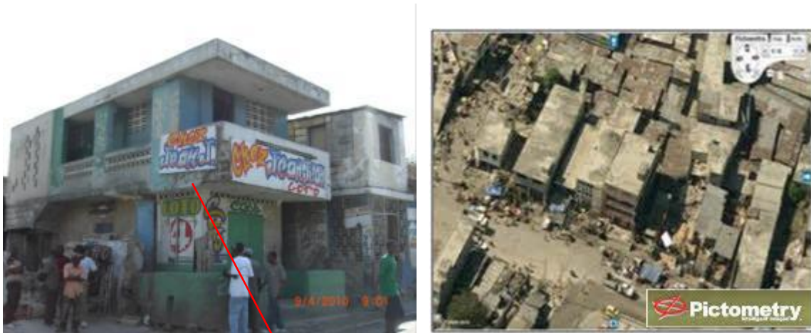
Figure 6.8: Typical buildings found in the commercial district in Port-au-Prince, long in one direction and rectangular in shape. (left) buildings seen from the ground, (right) buildings seen from above in Pictometry images (oblique aerial photos).
