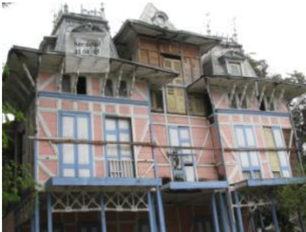
(a) Front façade
