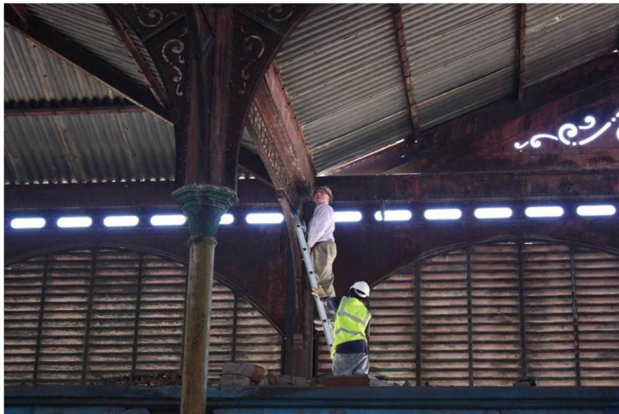
Figure 7.7: Internal view of south market, looking towards the south end
