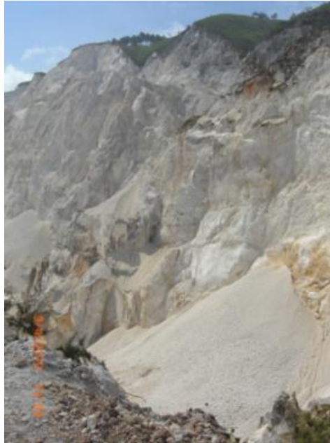
Figure 5.6: Localised landslides within the sand quarry
