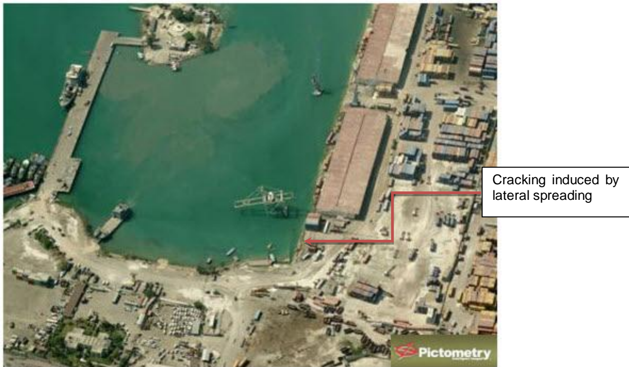
Figure 4.4: A Pictometry image of the overview of the collapsed north wharf and the crane (February 2010)
