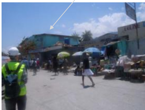
Figure 6.11: Ground view of building (a)
