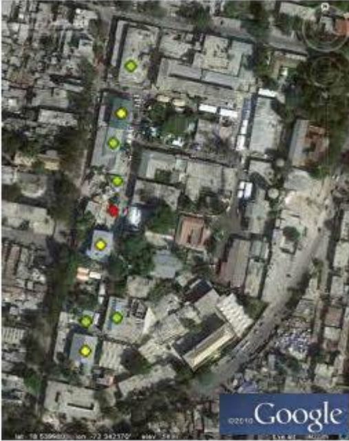
Figure 6.28: Overview of the buildings in location 55, surveyed by the EEFIT team.
