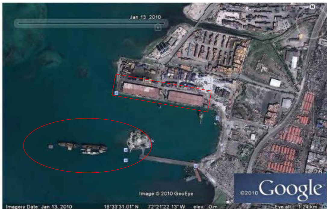
Figure 4.2: Post-earthquake satellite image of the port facility (13 th January 2010)
