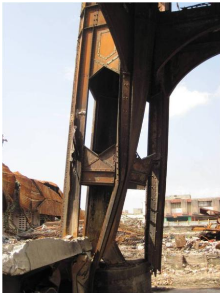
(a) Column base
