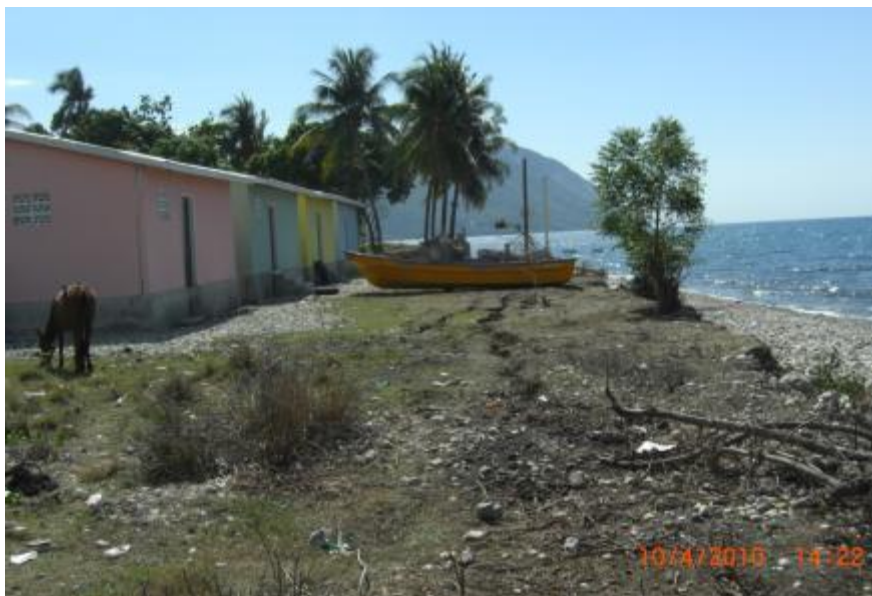
Figure 4.22: Evidence of lateral spreading close to the buildings
