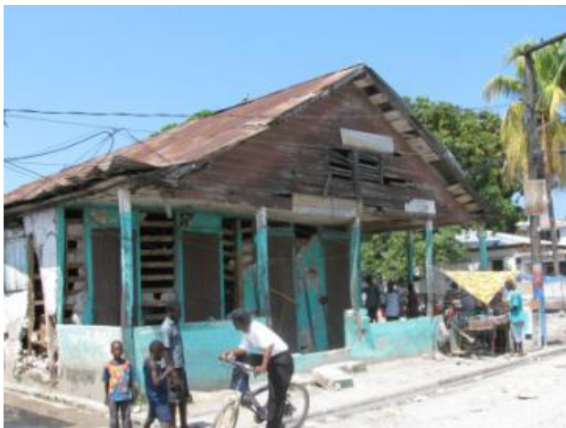
Figure 7.15: Single storey timber and masonry (colombage) building in Léogane
