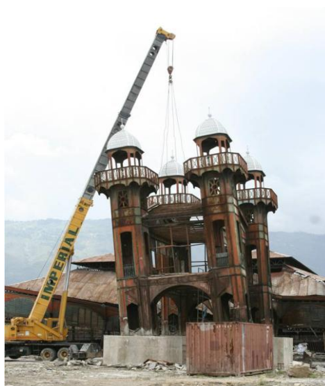
Figure 7.13: Refurbishment of the clock tower
