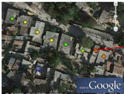
Figure 6.20: Overview of location 22 and the EEFIT damage grades.
