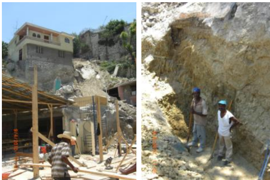
(a) Overview of failure (b) Excavation near base of slope
