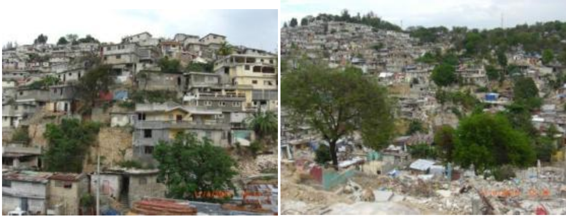
(a) Light damage
