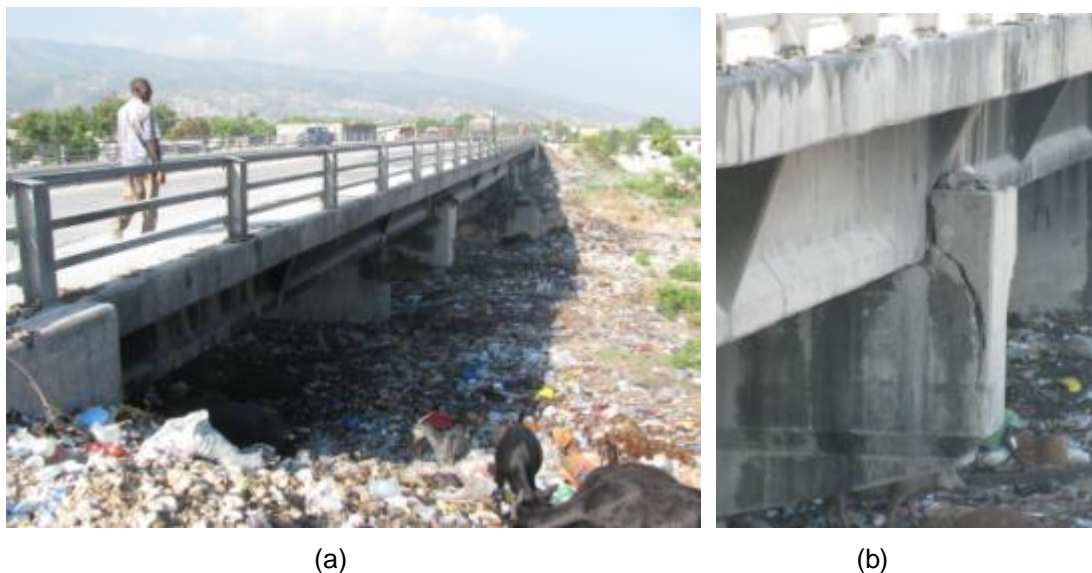
Figure 7.16: Bridge at Lemartin west of Port-au-Prince, near Carrefour
