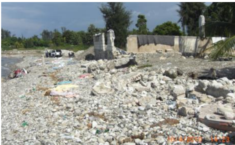
Figure 4.25: Collapsed building adjacent to laterally spreading ground
