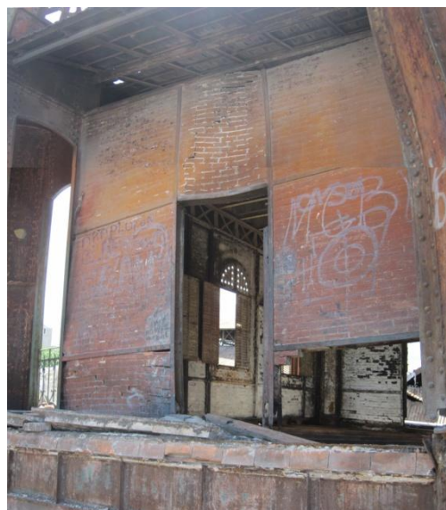
(b) Performance of infill masonry spandrels (composite of two photos)
