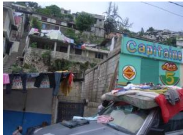
Figure 6.18: Buildings almost intact in location 17, although built on a steep slope.
