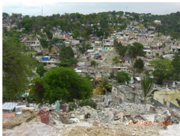
Heavy damage a few hundred metres away
