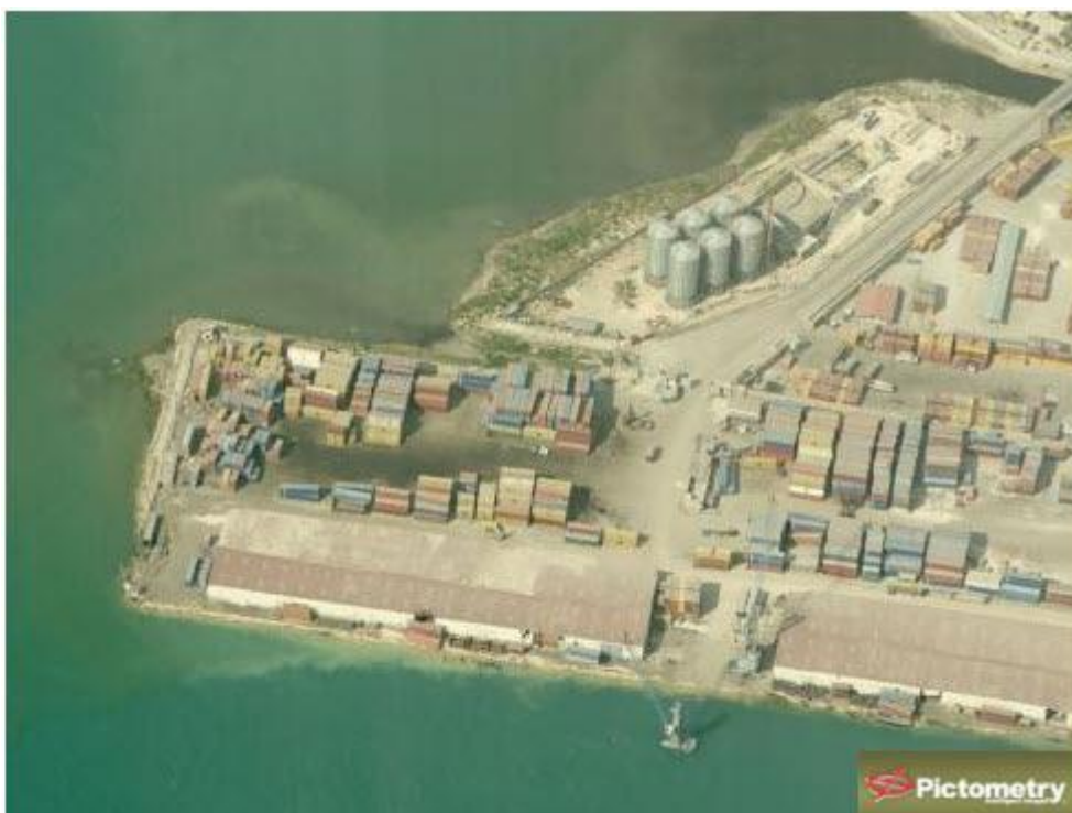
Figure 4.5: A Pictometry image of the mobile crane, container storage area behind north wharf and the silo structures (February 2010)
