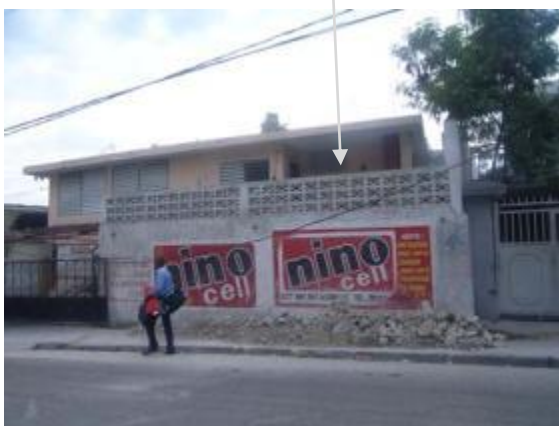
Figure 6.14: Building (a) which looks intact from the outside. EEFIT team did not have access to the premise. The aerial photo of the same building in Figure 6.13 shows some disturbance on the roof. Both Pictometry and GEO-CAN assigned D4.
