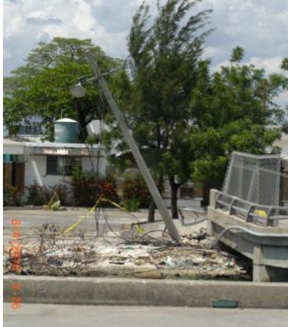
Figure 4.13: Lateral spreading causes an electricity pole to rotate
