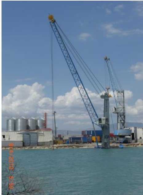
Figure 4.7: Damaged mobile crane at the time of the EEFIT visit
