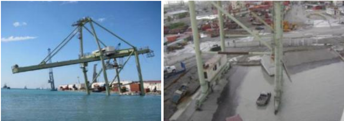
Figure 4.6: Collapsed gantry crane (Photos: Courtesy of Prof El-Gamal, UC San Diego)
