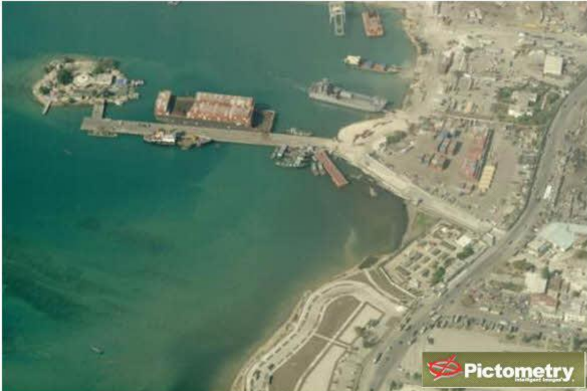
Figure 4.3: A Pictometry image of the overview of the south pier and the island (February 2010)
