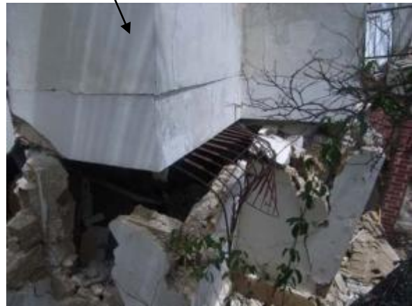
Figure 6.31: (left) Building under construction that suffered heavy damage, (right) soft storey building. Both buildings were assigned D5 by EEFIT, D5 and D4 by Pictometry, but were missed by GEO-CAN.
