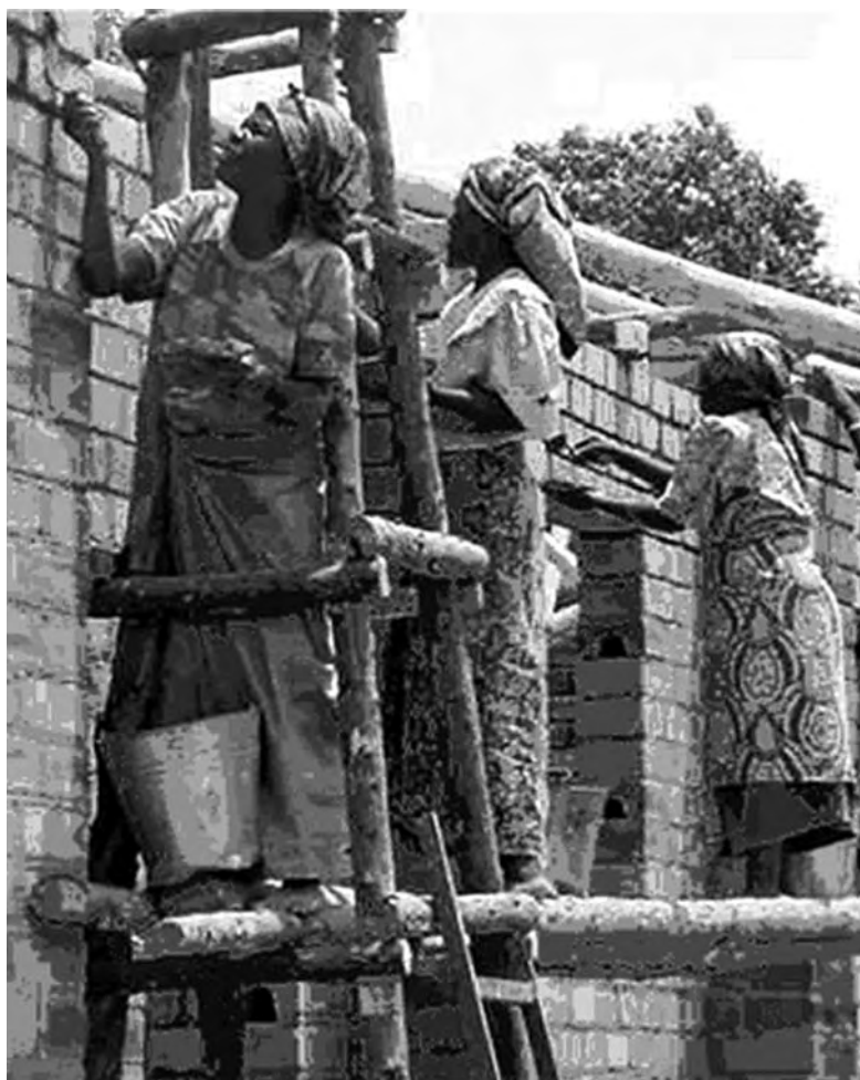
PHOTO 1 Women owner-builders in Huambo © Development Workshop
