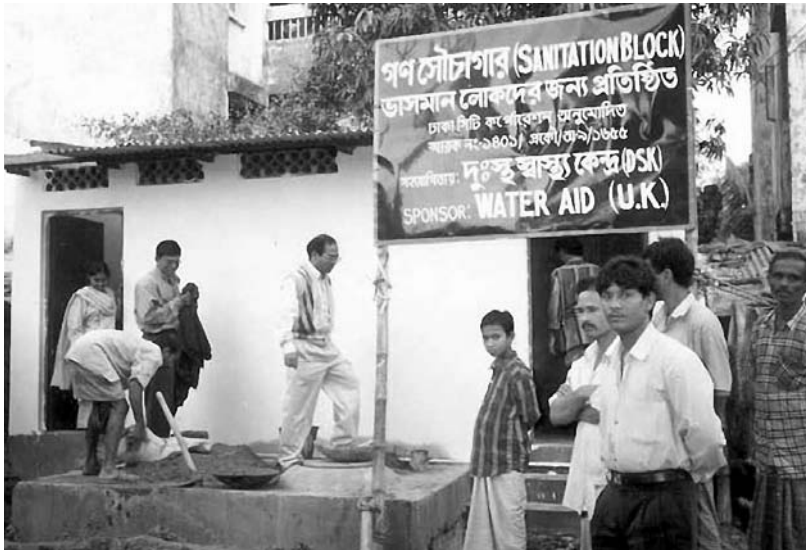
Photo 2: Sanitation blocks, which include latrine stalls, urinals and bathing space, are designed to serve up to 500 people
