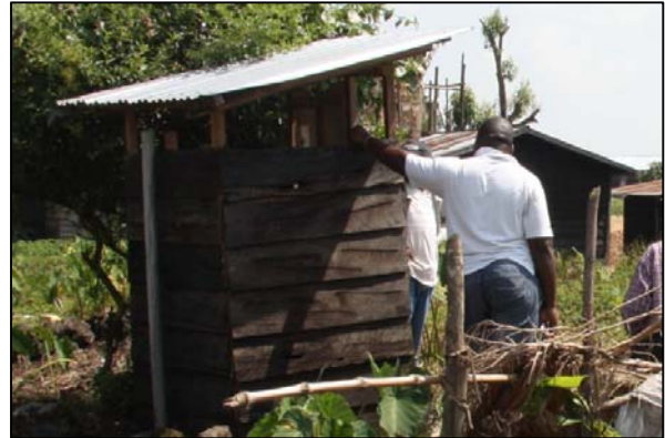
Picture 13. A family latrine in Kitchanga where the vent pipe is too short and covered by the roof, no fly screen is attached and too much light inside
