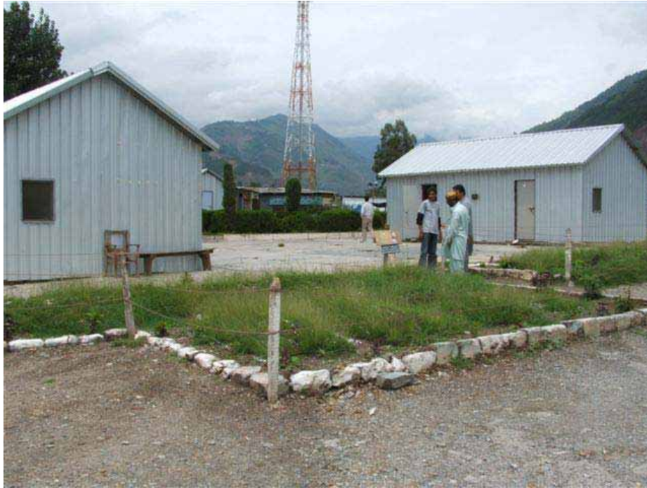
Figure 3: Temporary school buildings in Balacot where 150 students died when the school collapsed; 50 students remain permanently disabled. The grassy area in the foreground is a mass grave. The school previously catered for 750 students. The hill in the background previously accommodated a community of around 7,000 people; only 3,500 survived.
