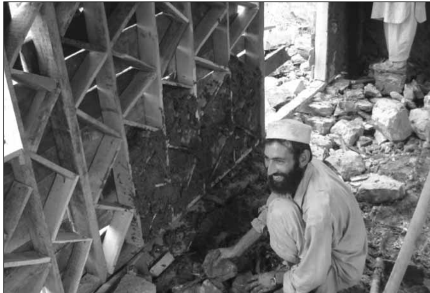
Figure 3.3 Reconstruction underway in Pakistan after the earthquake
