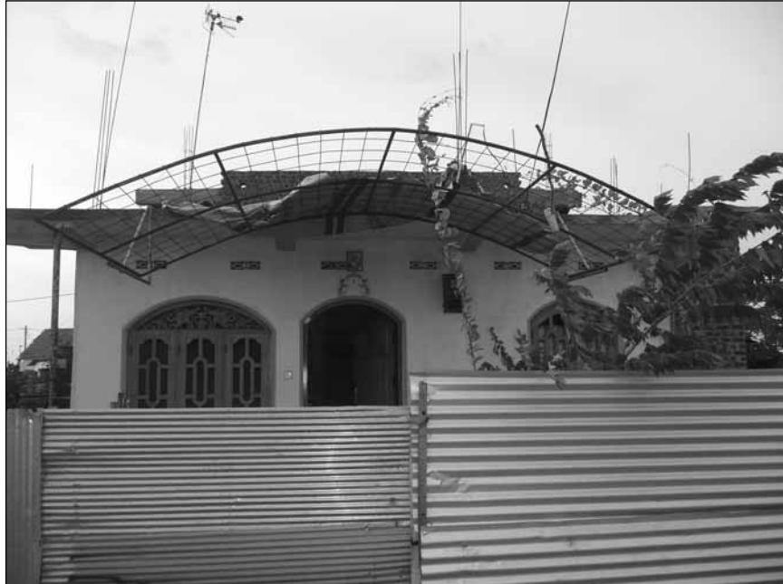
Figure 2.1 House 1: Flat-roof construction with ornamented windows and preparation for extensions
