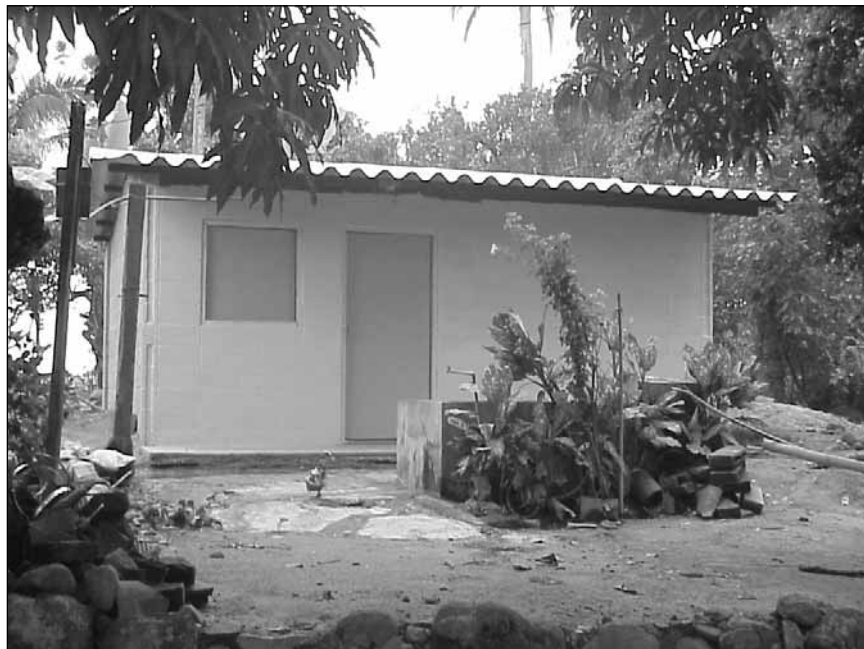
Figure 12.2 House painted at the end of stage two in San Antonio Jiboa
