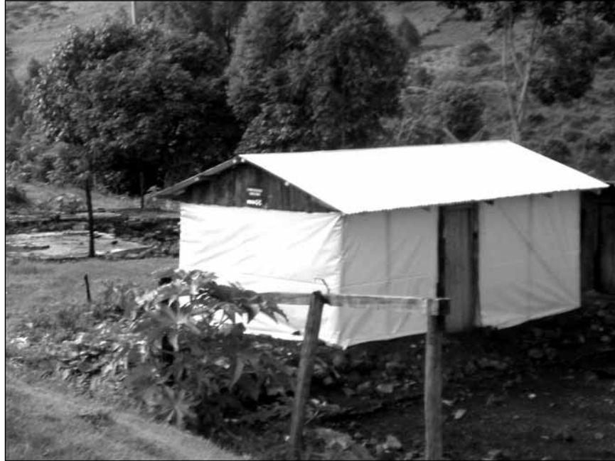
Figure 9.4 Shelter: Partial upgrade with reclaimed materials
