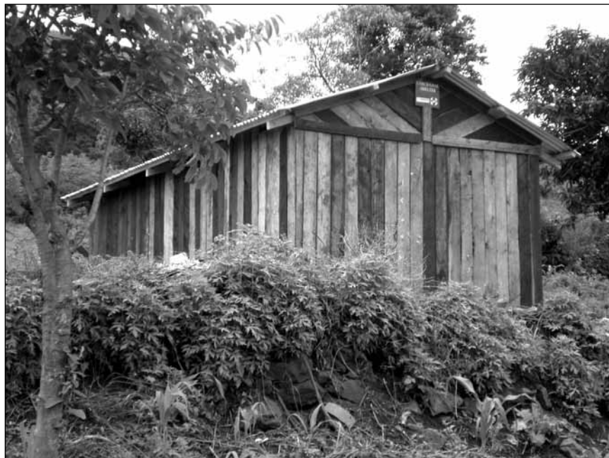
Figure 9.5 Shelter: Upgrade with timber off-cuts
