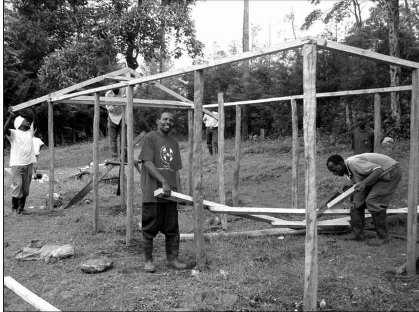
Figure 9.2 Assembling the frame
