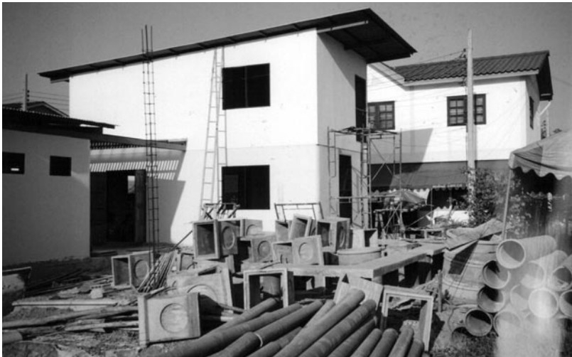
Photos 3 and 4: Klong Lumnoon, before land-sharing and during upgrading
