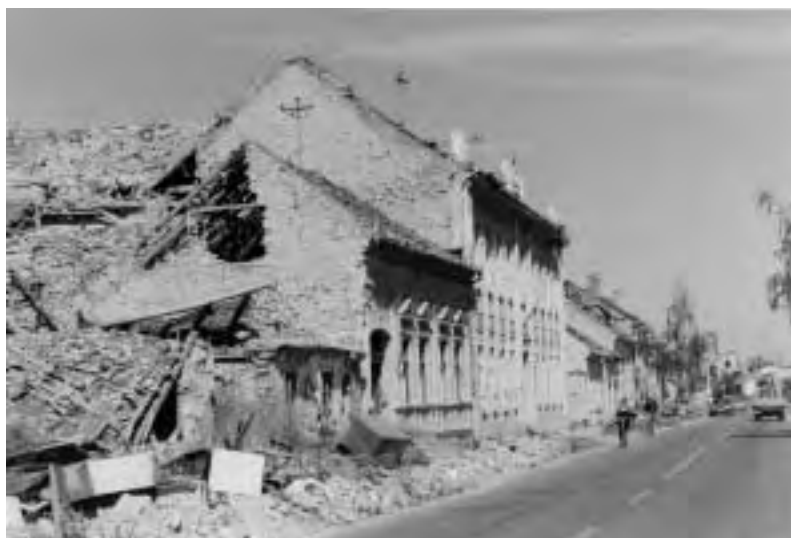
War-damaged homes, Vukovar, Croatia, September 1992
