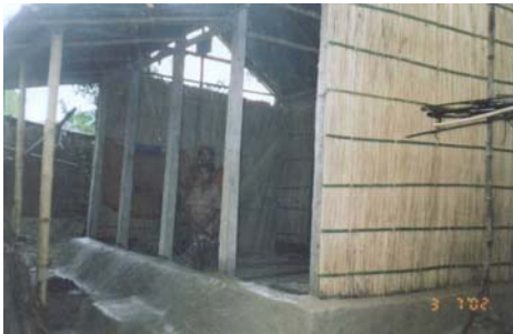
A house under construction
