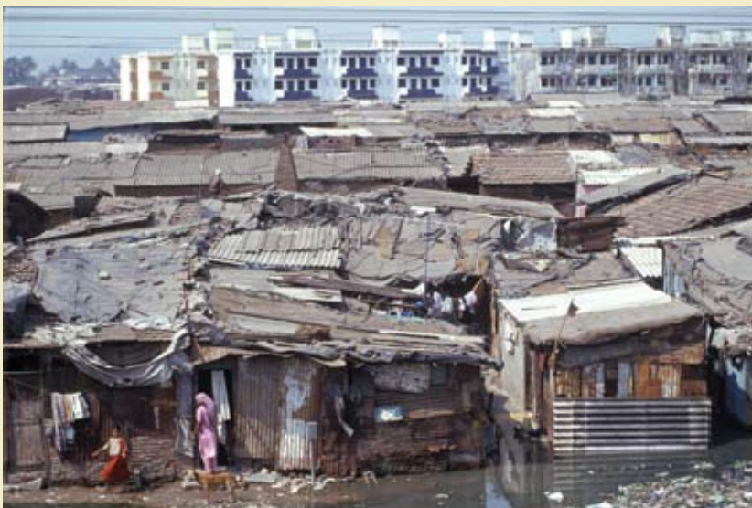
Waterlogged slum housing in Mumbai, India
