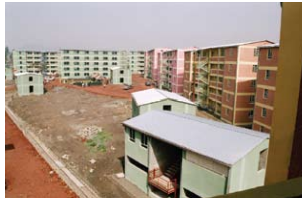
Newly constructed condominium houses under the Integrated Housing Development Programme, Addis Ababa, 2007.
