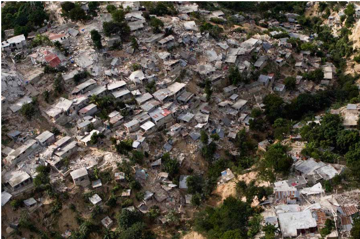
Fig. 4 Houses built on the slopes collapse into one of the ravines in Port au Prince. The land which the house occupied is essentially destroyed. Image: (UN, 2011c)
