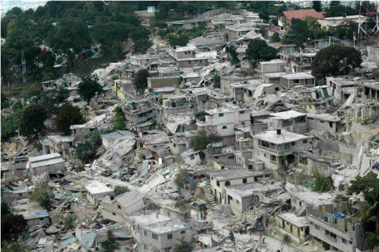
Fig. 5 A road through a neighbourhood in Port au Prince. Often access to individual buildings is via narrow pathways, as little as 3ft wide, which means that there is little spare land for the introduction of infrastructure and services. Image: (IFRC, 2011a)
