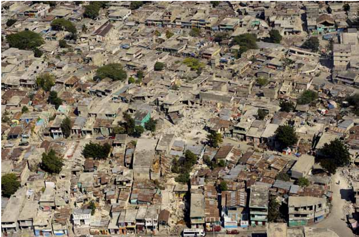
Fig. 14 Aerial view of collapsed buildings. Though most are low rise (1-3 storeys), the lack of space between buildings means that reconstruction on one site will inevitably impact on neighbouring sites. Image: (US Navy, 2011b)
