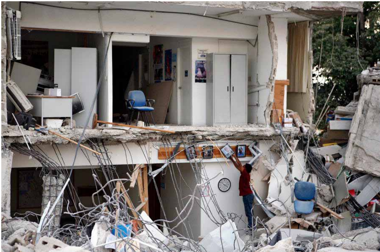
Fig. 6 The UN mission. A large number of public and institutional buildings were destroyed in the earthquake, including the Presidential Palace, Parliament and most of the Ministries (Govt. of Haiti, 2010). Image: (UN, 2011d).
