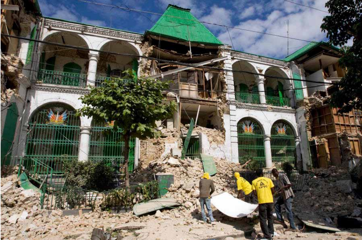
Fig. 7 The collapsed public works ministry. Image: (UN, 2011e)
