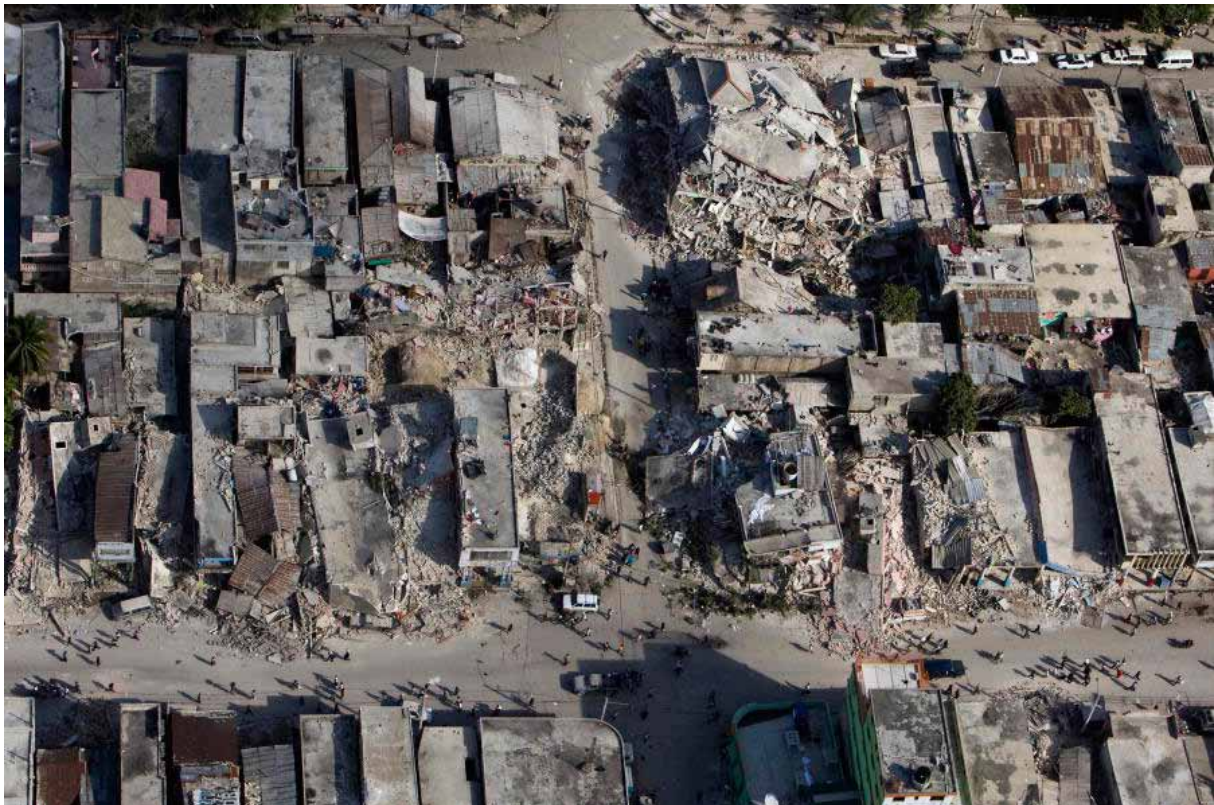
Fig. 3 Earthquake damage in the centre of Port au Prince. Image: (UN, 2011b)
