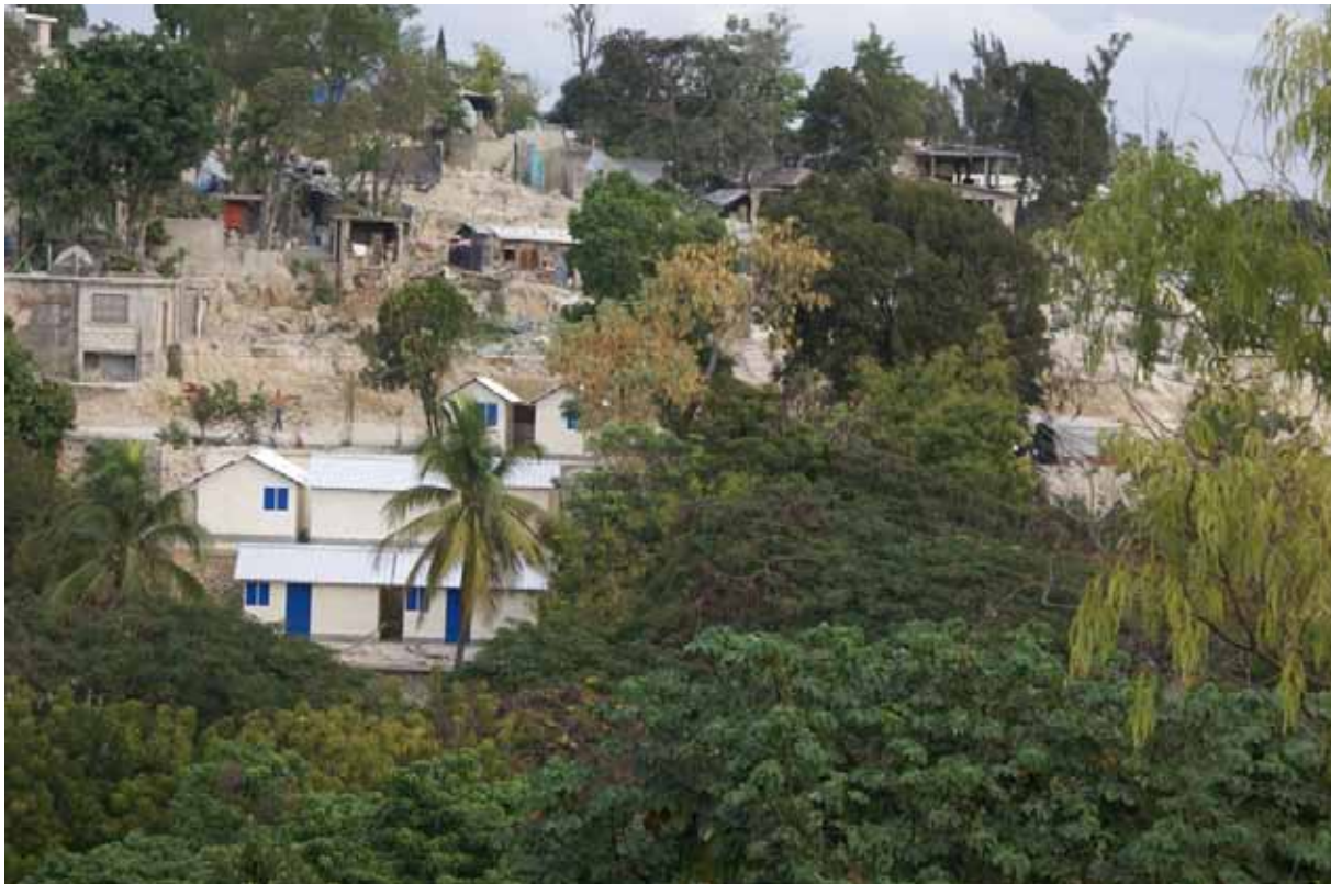
Fig. 16 Transitional shelters on one of Port au Prince's hillsides. They are designed as stand alone structures and cannot support the same densities as the pre-earthquake buildings. Image: (TSC Global, 2011)
