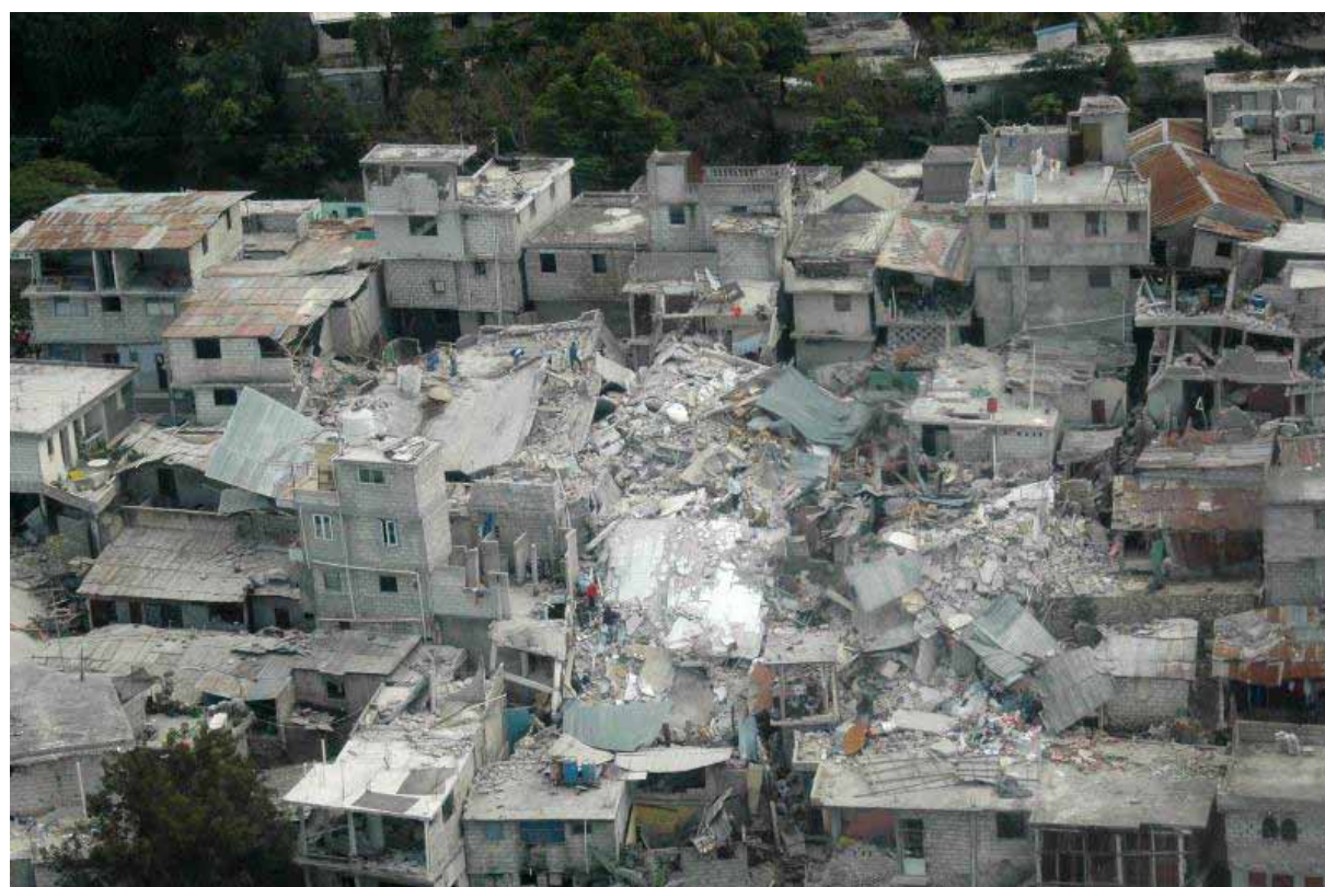
Fig. 15 A collapsed hillside in Port au Prince. The majority of buildings are between 1 and 3 storeys and share party walls. Sites are densely occupied. Image: (IFRC, 2011b)
