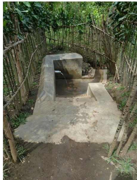
Figure 4 Protected spring of good quality
