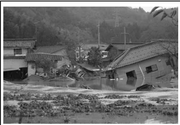
Houses near the dike were severely damaged or destroyed
