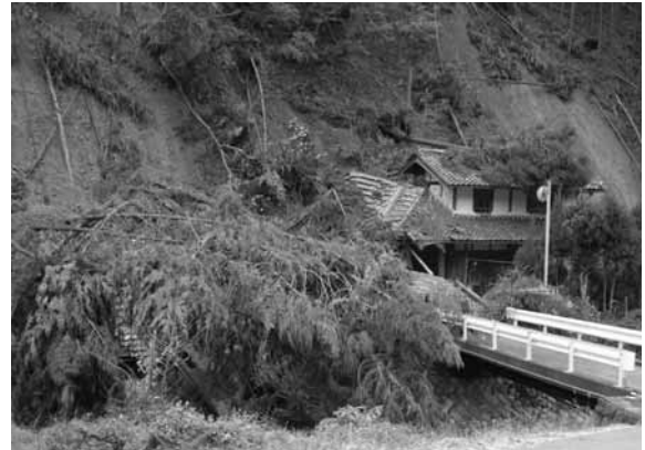
Damaged of landslides
