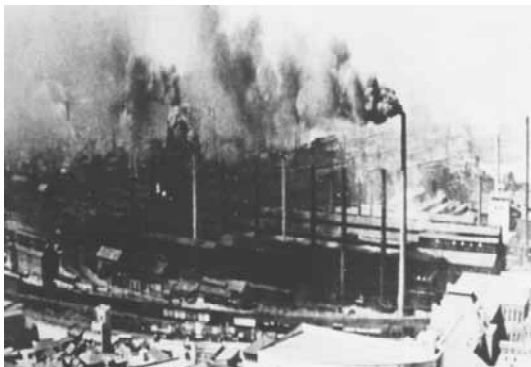
Smoke Emitted from Chimneys
