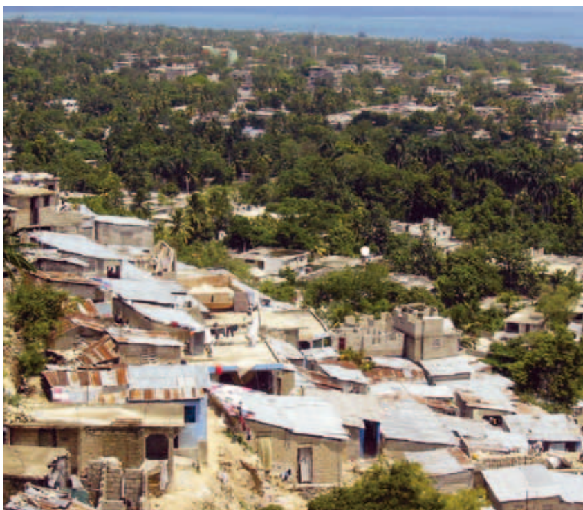
In Port-au-Prince, it is common to build on landslide prone areas Photo © Å. Forsman
