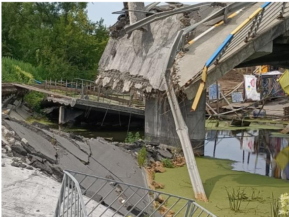
Irpin bridge, destroyed at the beginning of the war
