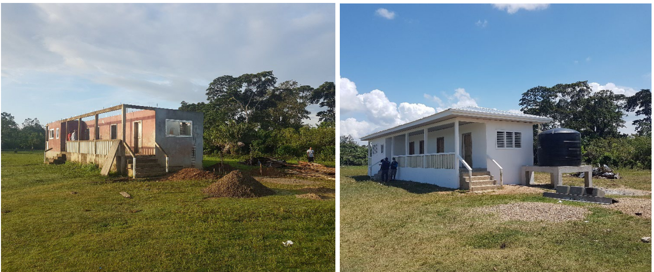
Lakunka health facility: before and after repairs
