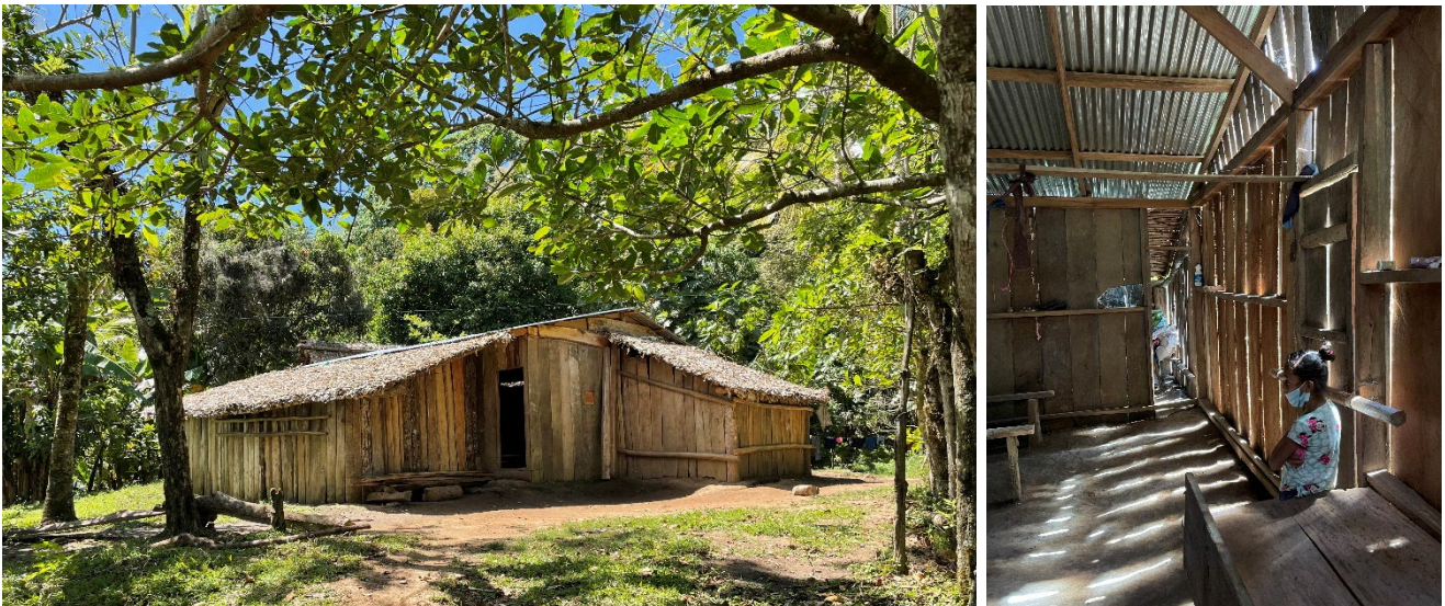
In some cases, the zinc was used to cover the main house and annex buildings are covered with leaves
