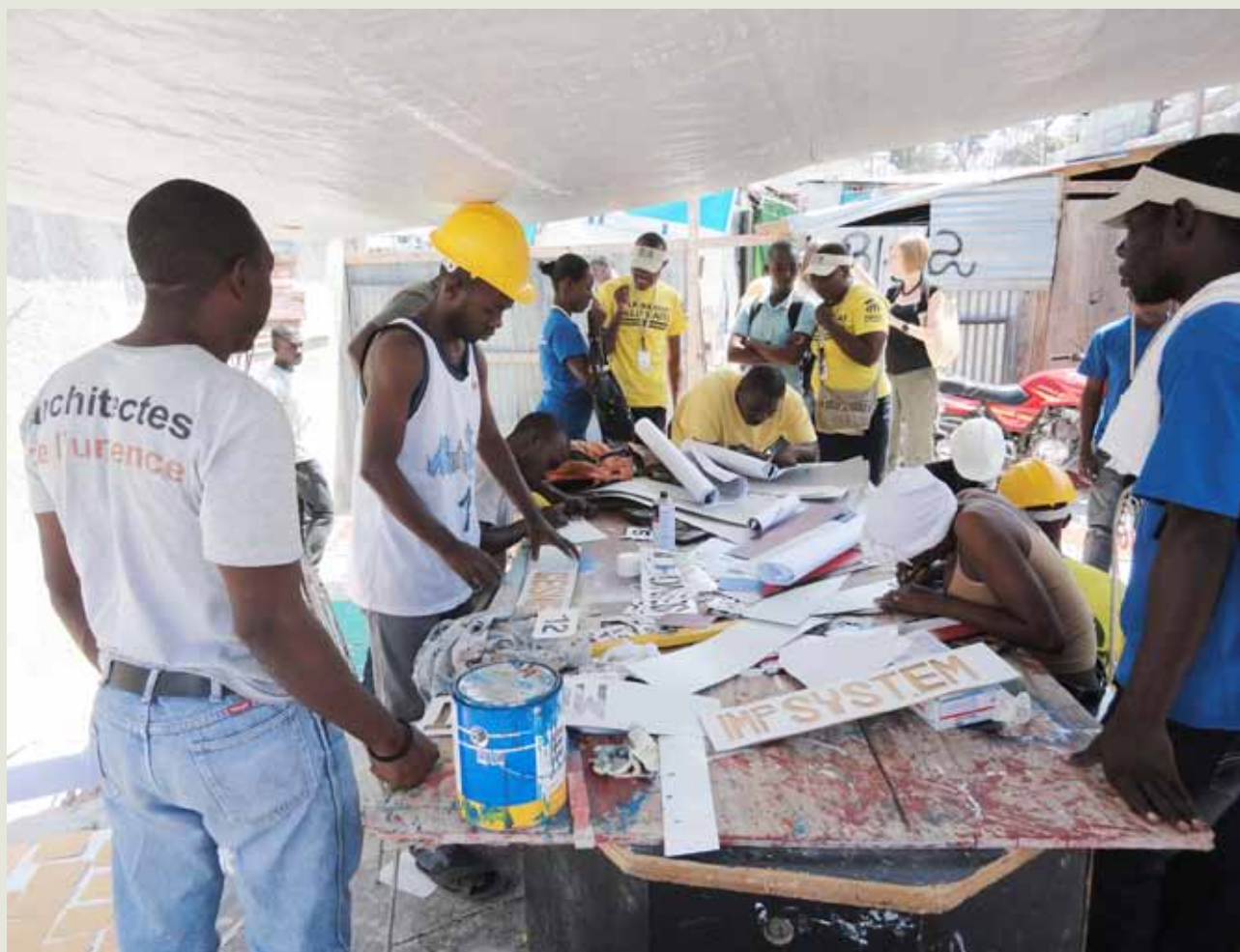
Bristout-Bobin, Haiti. UN-Habitat reconstruction project in collaboration with Fondation Architectes de l'Urgence. © UN-Habitat/FAU
