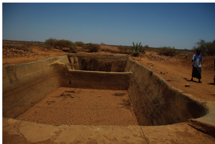
The Berkad at Burtinle showing poor design the resultant heavy silting
