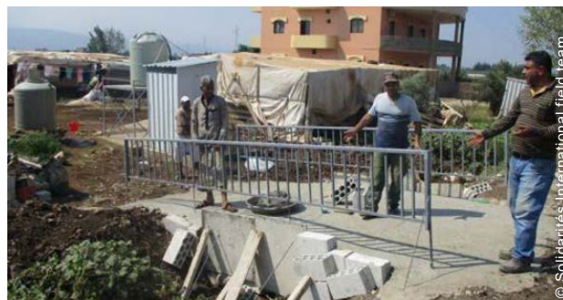
Accessibility interventions in Informal Tented Settlements included improving wheelchair access.
