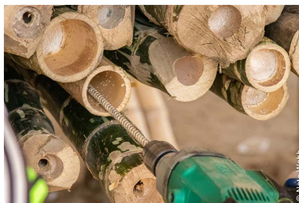
Bamboo for construction is mostly supplied from Rangpur in the north of Bangladesh.
