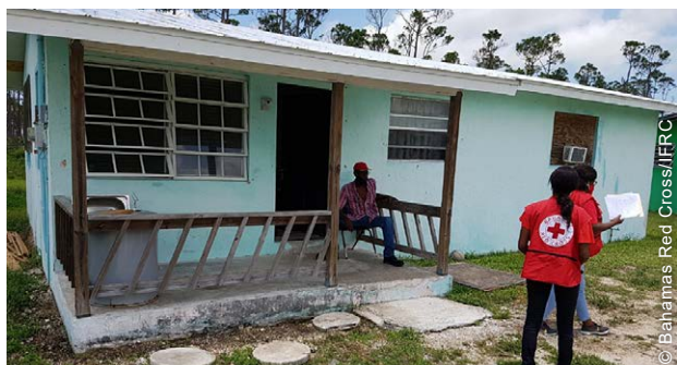
Homes outside of Freeport, the main city on Grand Bahama, are typically timber framed or concrete block single story structures.
