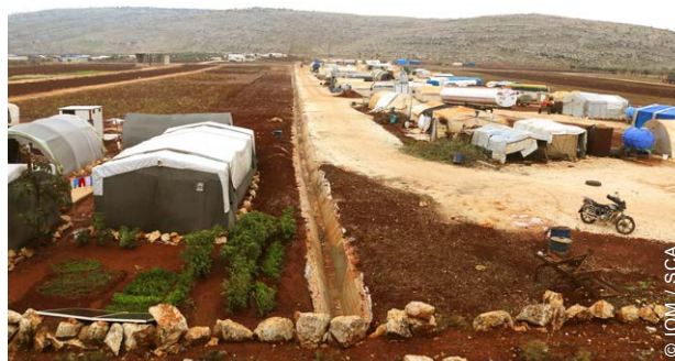
After: An informal camp, post-flood mitigation intervention.
