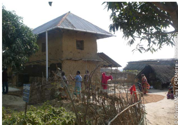
This low-cost housing project in Bangladesh provides families with core houses which are then completed through safe self-build practices in progressive or incremental stages as a crucial step of self-recovery.
