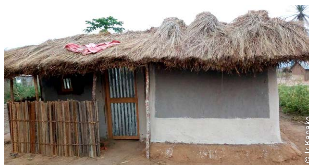
In the Democratic Republic of the Congo, this project included verandas for cooking in order to reduce health and fire risks. For more information see Shelter Projects 2017-18 (A2) p7 .
