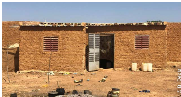
Semi-durable shelter made of mud brick. IDPs are supported with technical guidance and cash for these constructions.
