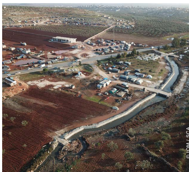
Storm drainage channels were a key site improvement intervention to mitigate the risk of flooding.
