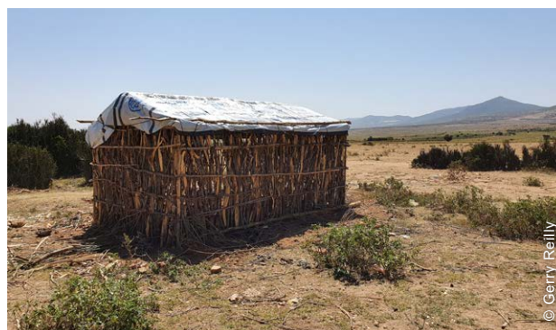
Plastic sheeting distributed in the first installment was used as a temporary roofing material prior to households receiving the second installment.
