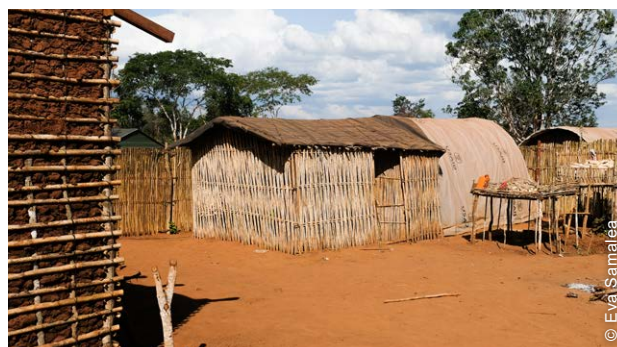
Shelter phased approach development by one household in Meculane Relocation Site, Chiure, Cabo Delgado.
