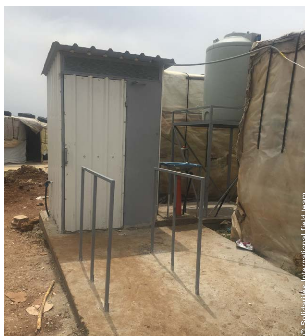
Accessibility of latrines in informal tented settlement was improved.
