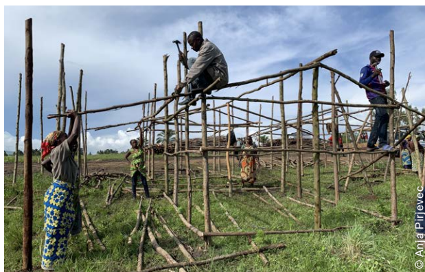
Special effort was made to involve women in the construction teams.
