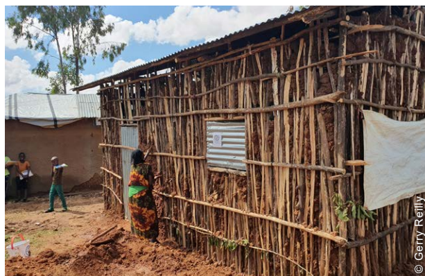
The main shelter typology in East Hararghe is typically a wooden structure that consists of wooden poles harvested locally, wooden infill from wild bushes, and mud plastered walls.
