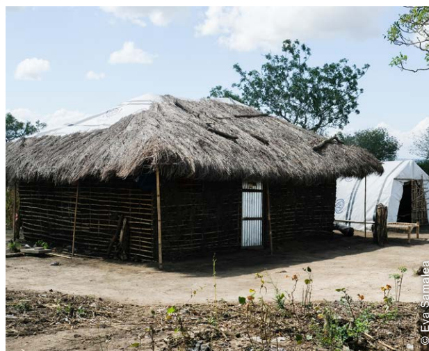
Emergency Shelter and Semi-Permanent Shelter (self-built) as part of the upgrade strategy within the same household, Ntokota Relocation Site, Metuge, Cabo Delgado.
