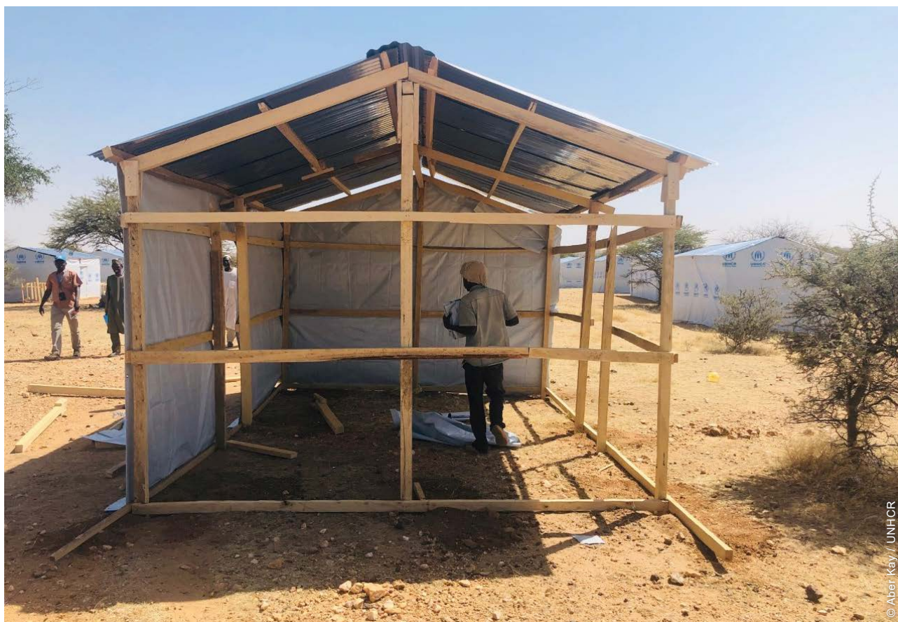
Temporary family shelters were constructed for each refugee household arriving at the new settlement. The intention was that the shelter walls could later be upgraded by households by using more resilient locally available materials such as wattle and daub.
