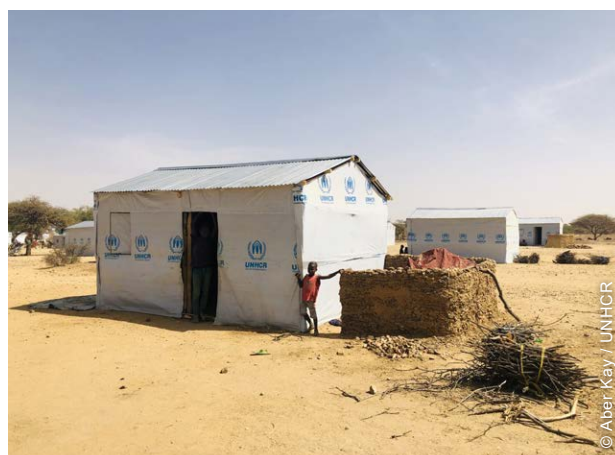
Some families already commenced with the construction of other shelters within their plot for kitchens or to use as an extra room using locally available materials of stones, mud, wattle and thatch.
