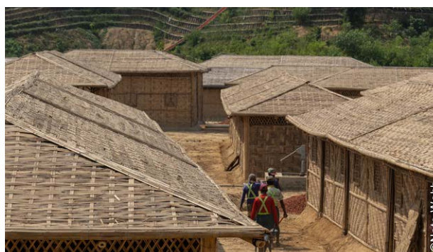
Mid-Term shelters were constructed in the valley areas.
