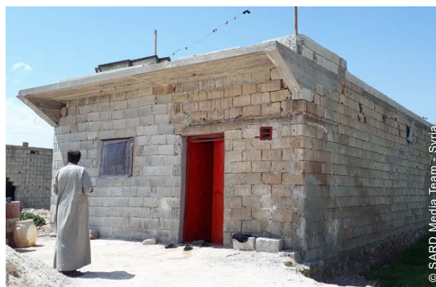
Before and after photos showing house rehabilitation.
