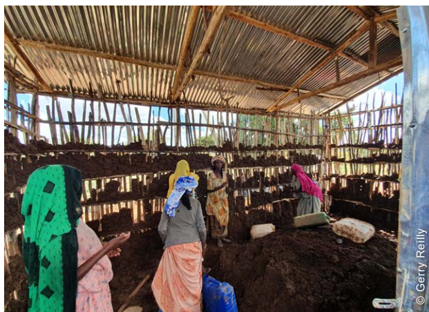
Each group of 12 households were responsible for progressing all the group's shelters in order for the group to collectively qualify for the next stage of assistance. The image above shows a group of women carrying out mud plastering.
