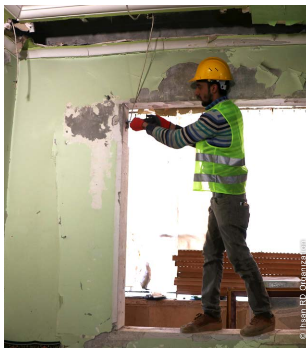
Upgrades of building elements such as doors and windows to ensure that buildings were better sealed off greatly improved winterization and protection.
