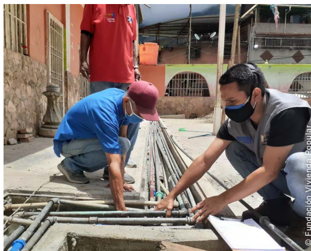
Community-level interventions included the rehabilitation of water pipelines.
