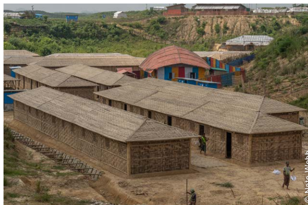
The newly constructed shelters provided accommodation to families who were being relocated from other areas of the camp that were congested or faced disaster-risk.
