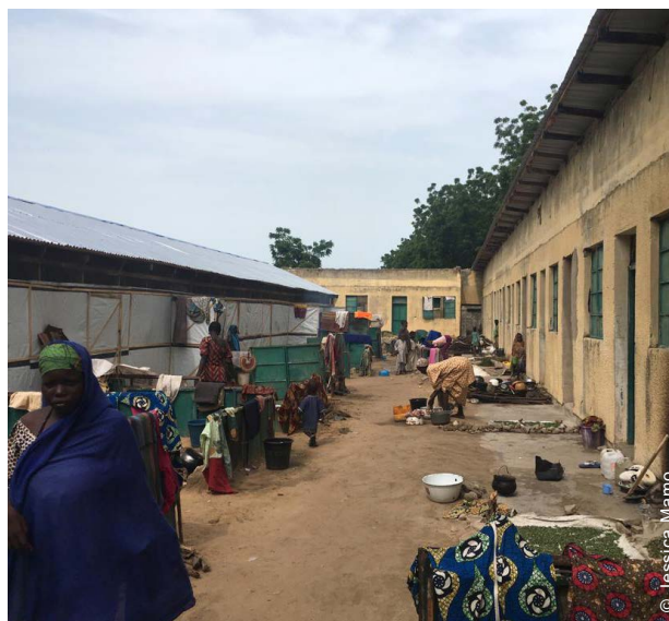
Existing buildings on the site were rehabilitated and partitioned (right) to provide additional shelter in the camp. Partitioned communal shelters (left) were also constructed due to the lack of space for individual family shelters.
