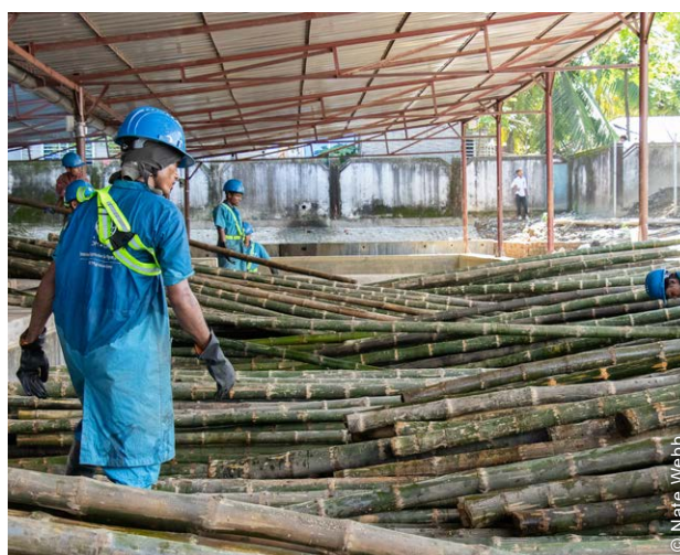
The facility has a daily production capacity of treating 2,500 bamboo poles.
