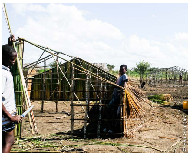
Support was provided to households building their own shelters using locally available materials. This included trainings and awareness raising on more resilient construction techniques, and on mitigation of the potential negative environmental impacts of shelter construction.
