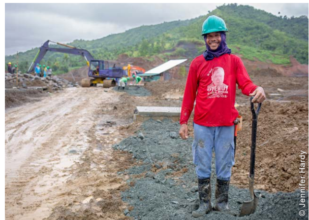
Local workers were engaged through small construction contractors for the Site Development of DREAMville and were supervised by the organization's technical team.
