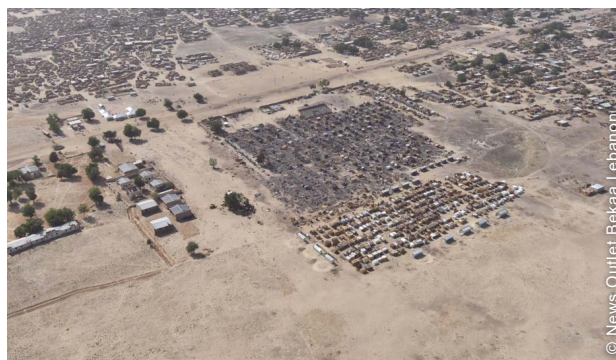
Fire damage from a February 2019 fire at Monguno Camp in Borno State, Nigeria, where multi-fatality fires have frequently harmed affected populations, destroyed IDP camps and undermined humanitarian assistance.
