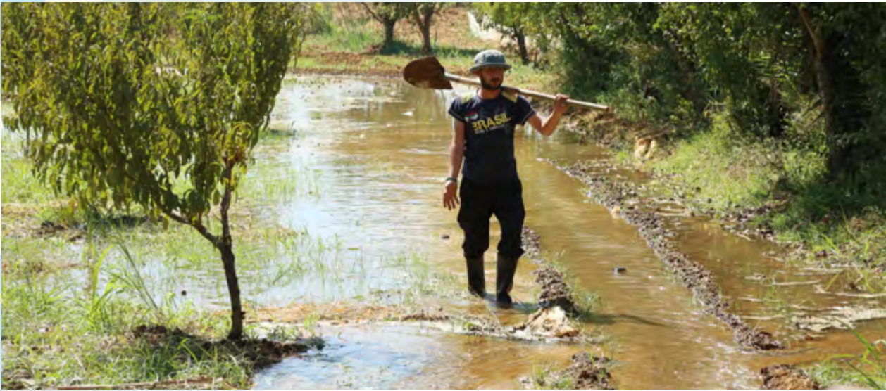
Figure 19- Construction of an irrigation canal in Qabb Elias. Photo credits: UNDP, 2016.
